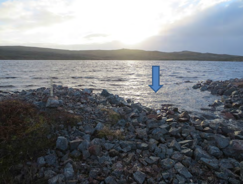
View upstream towards Pond
