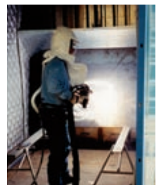
Thermal/Flame Spray After Gold Series® Turned On
