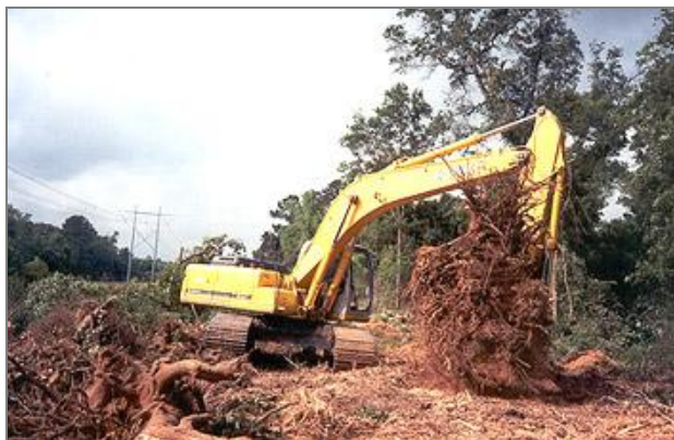
Figure 10-12 - Example of Grubbing Activities
