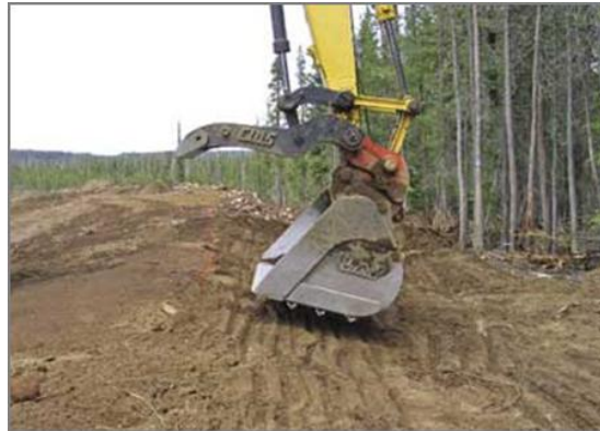
Figure 10-20 - Photograph of Grooving Slope Treatment Method
