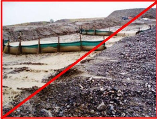
Figure 10-22 - Examples of Poorly Installed Silt Fences
