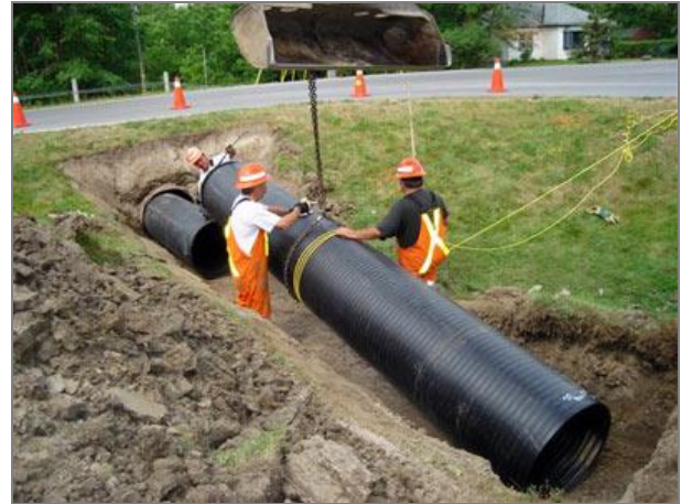
Figure 10-8 - Example of Culvert Installation
