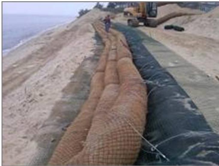
Figure 10-124 - Photograph of Fibre Rolls used to Stabilize
