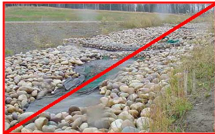
Figure 10-157 - Photograph of failed Rip Rap Protection a Slope
