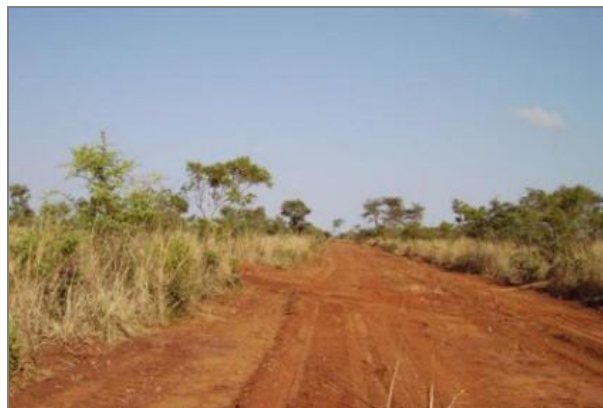
Figure 10-23 - Example of Grubbed and Cleared Path
