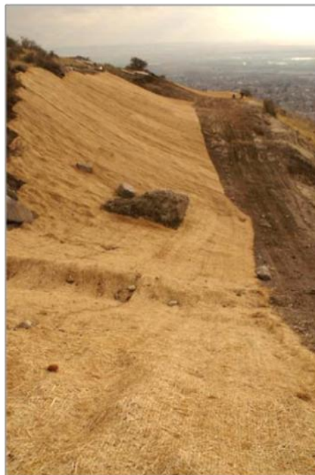
Figure 10-113 - Photograph of Erosion Control Blanket used on a Slope
