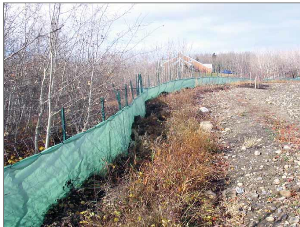
Figure 10-9 - Tarp Fence Outlining a Vegetation Buffer Zone
