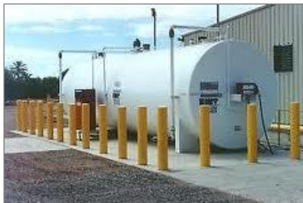
Figure 10-6 - Fuel Storage on Concrete Pad
