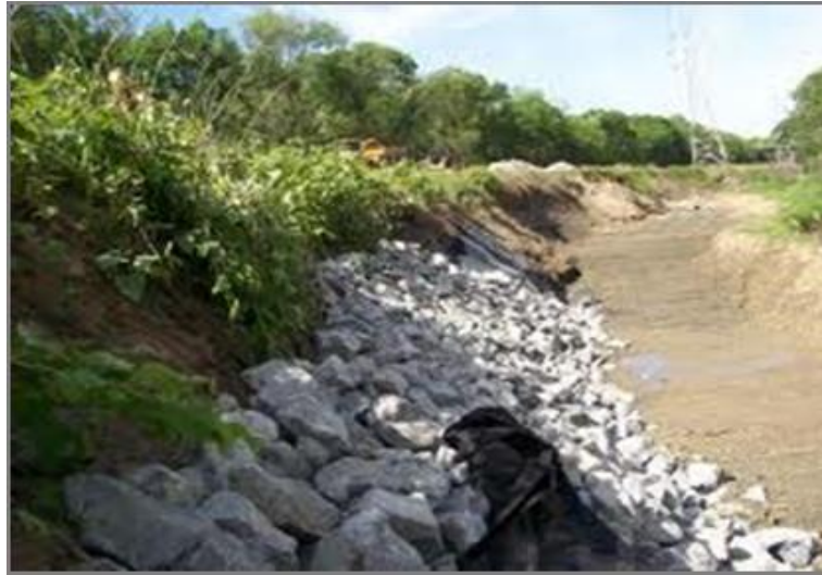
Figure 10-146 - Photograph of Rip Rap Placed Along a Slope
