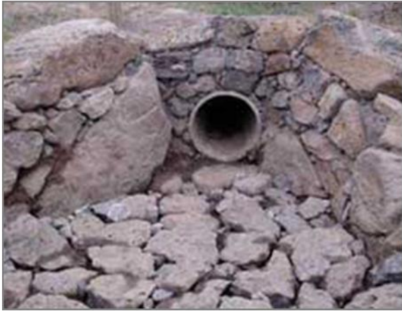
Figure 10-18 - Correct Construction of Rock Energy Dissipaters
