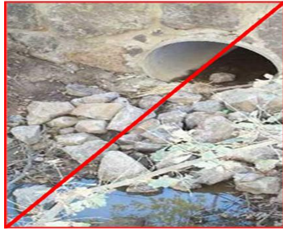
Figure 10-31 - Incorrect Construction of Rock Energy Dissipaters
