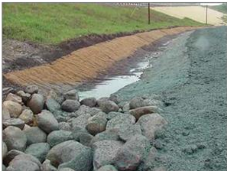
Figure 10-135 - Photograph Shows Erosion Control Blanket on Slope And Erosion Control Mat in Channel
