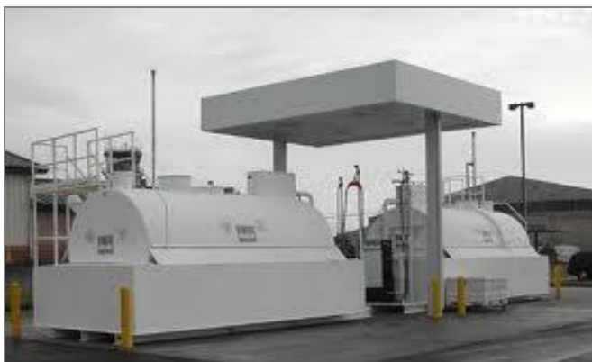
Figure 10-5 - Acceptable Fuel Storage with Dykes
