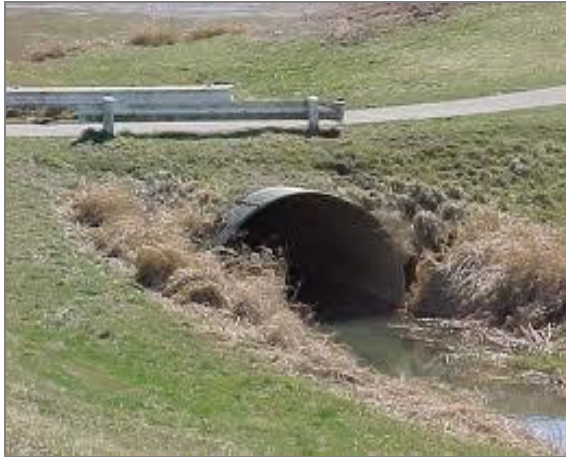
Figure 10-7 - Example of Well Installed Culvert
