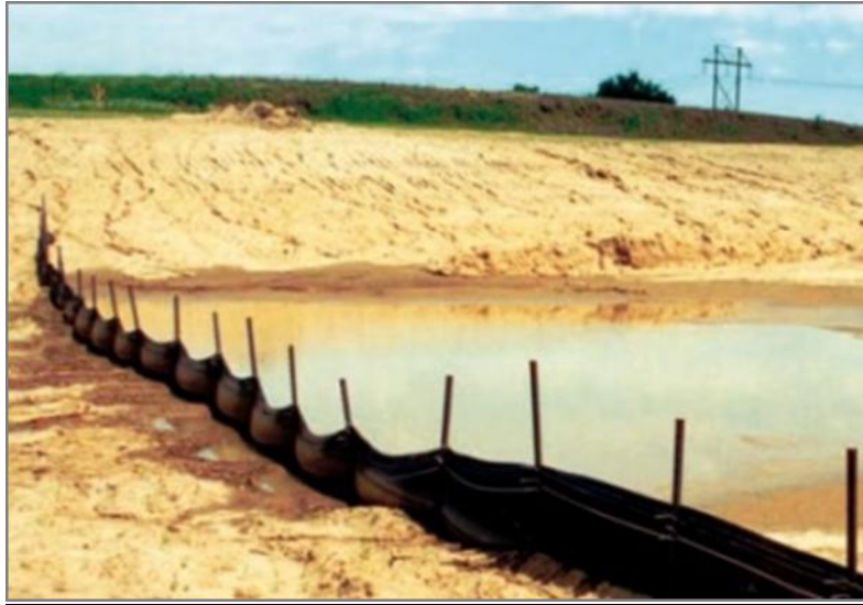
Figure 10-19 - A Well Constructed Silt Fence
