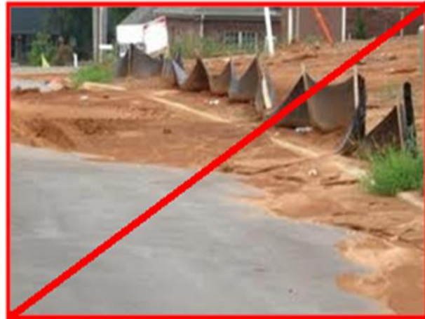
Figure 10-23 - Examples of Poorly Installed Silt Fences
