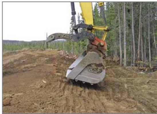
Figure A-1 - Photograph of Grooving Slope Treatment Method
