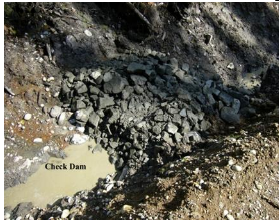
Figure A-9 - Photograph of Rock Constructed Check Dam
