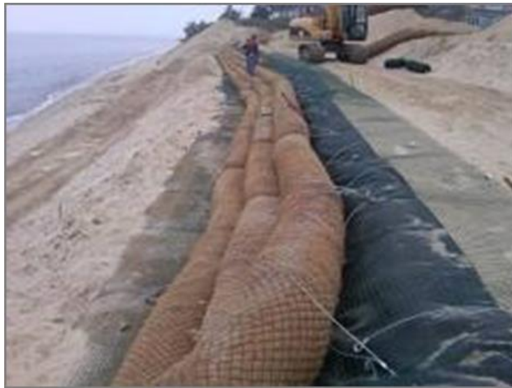
Figure A-5- Photograph of Fibre Rolls used to Stabilize
