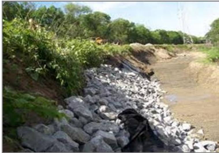
Figure A-7- Photograph of Rip Rap Placed Along a Slope
