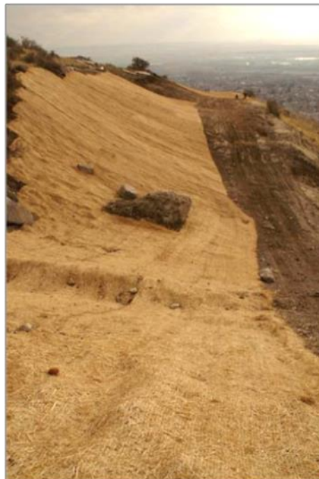
Figure A-4 - Photograph of Erosion Control Blanket used on a Slope
