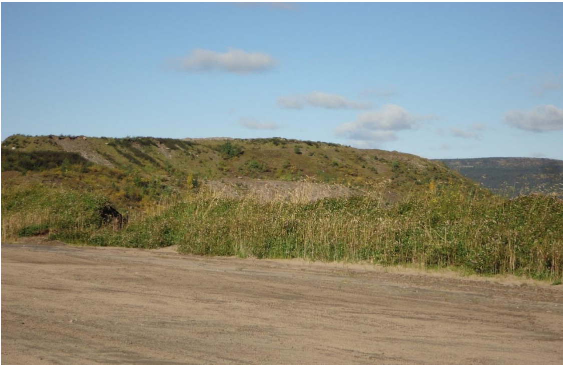
Waste Rock Dump #11 Facing North
