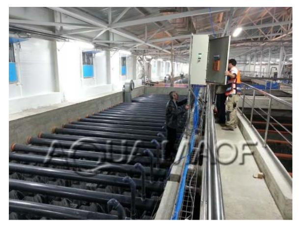
Biofilter spray nozzles distributing water over media of the trickling filter in a trout production facility. Note the air blower for CO2 degassing at middle left side of biofilter. Multiple blower fans supply water to an air space below the media stack. Technicians adjusting the controls for water flow to the biofilter nozzles. View of the tube settler on the far right that supplies water to the nozzles with gravity flow.
