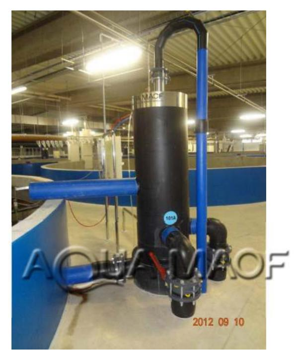
AquaMaof oxygen dissolving system (ODS) showing duplicate water supply from the pipes on lower portion. The duplicate water supply pipes are connected separately to duplicate water pumps. The pipe extending to the top is for adding new water as required. Oxygenated water flows from the ODS through the tank sidewall. The pipe extending from the ODS over the tank sidewall is an overflow pipe.
