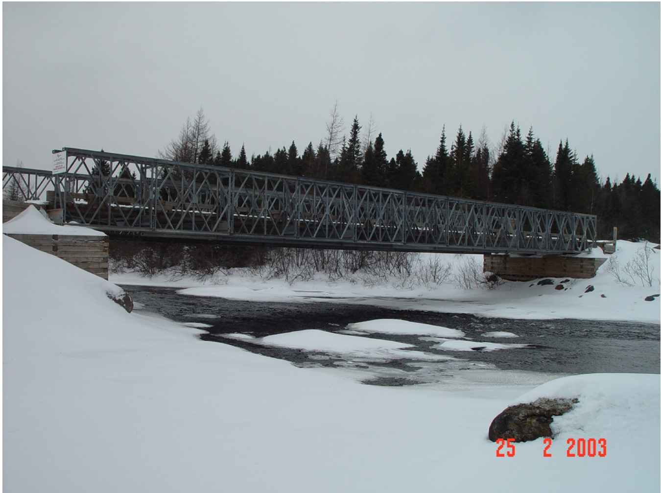
Figure 2.2 Photograph of Noel Paul's Brook with a Temporary Bailey Type Bridge in Place in 2003
