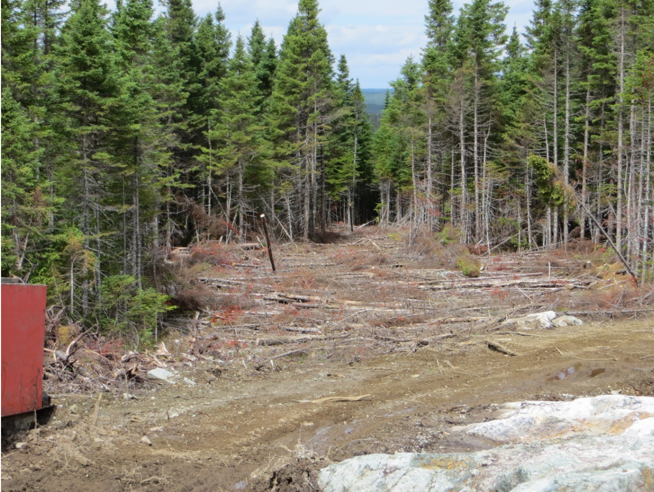
Plate 5: Example of drill site reclamation involving smoothing and contouring of overburden, then covering by organic layer, felled trees and brush as well as highway-blend grass seed.
