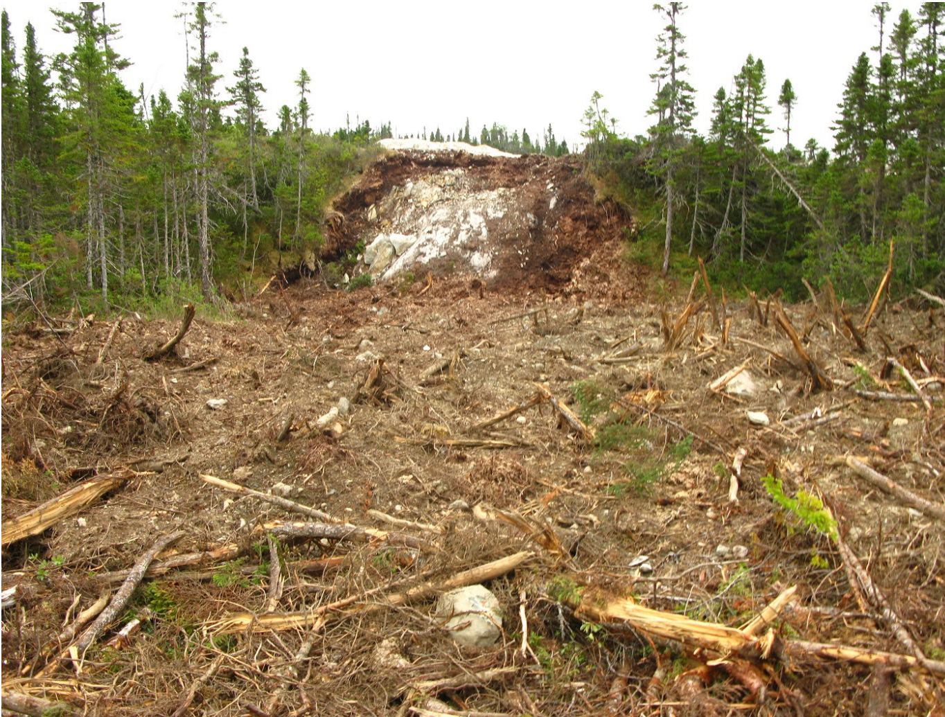
Plate 9: An example of a partially backfilled trench showing smoothed surface covered with till, organics and grass seed.
