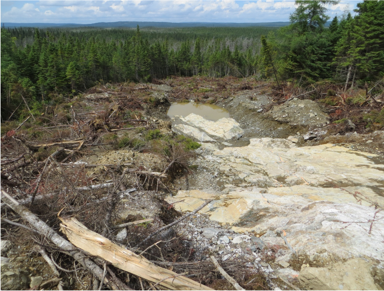
Plate 8: Example of stockpiled organic material and till set aside for later backfilling and reclamation of trench.
