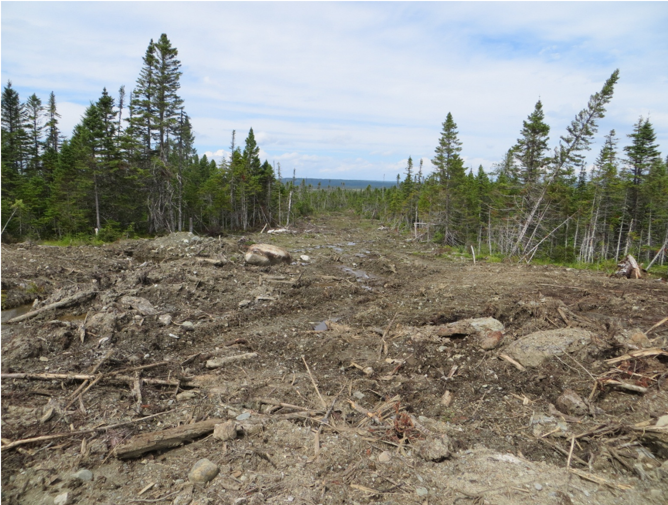
Plate 2: Example of drill access skidder trail reclamation involving leveling of ground disturbance followed by contouring of overburden and covering by organic layer as well as hay and highway-blend grass seed where limited organics.
