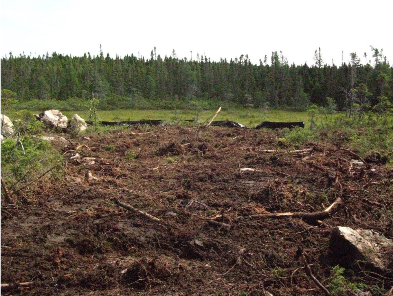
Plate 6: Example of drill site reclamation involving smoothing and contouring of overburden, then covering by organic layer and brush as well as highway-blend grass seed. Note silt screen along edge of wet area to prevent siltation runoff into boggy area.
