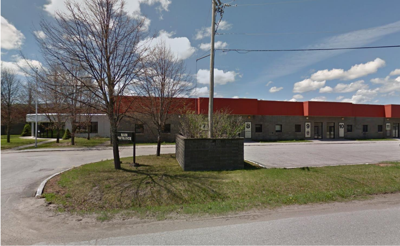
Exhibit 4 – Street View of Pardy’s Venture Centre
