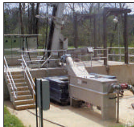
The Helisieve Plus® Septage Receiving Station turns plants into professional receiving stations overnight
