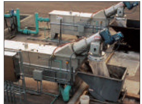
Two septage receiving stations set up as income producers for a private enterprise
