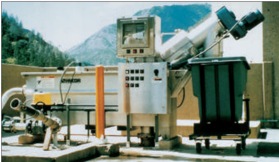
User-friendly, maintenance-free septage pre-treatment protects downstream processes.
