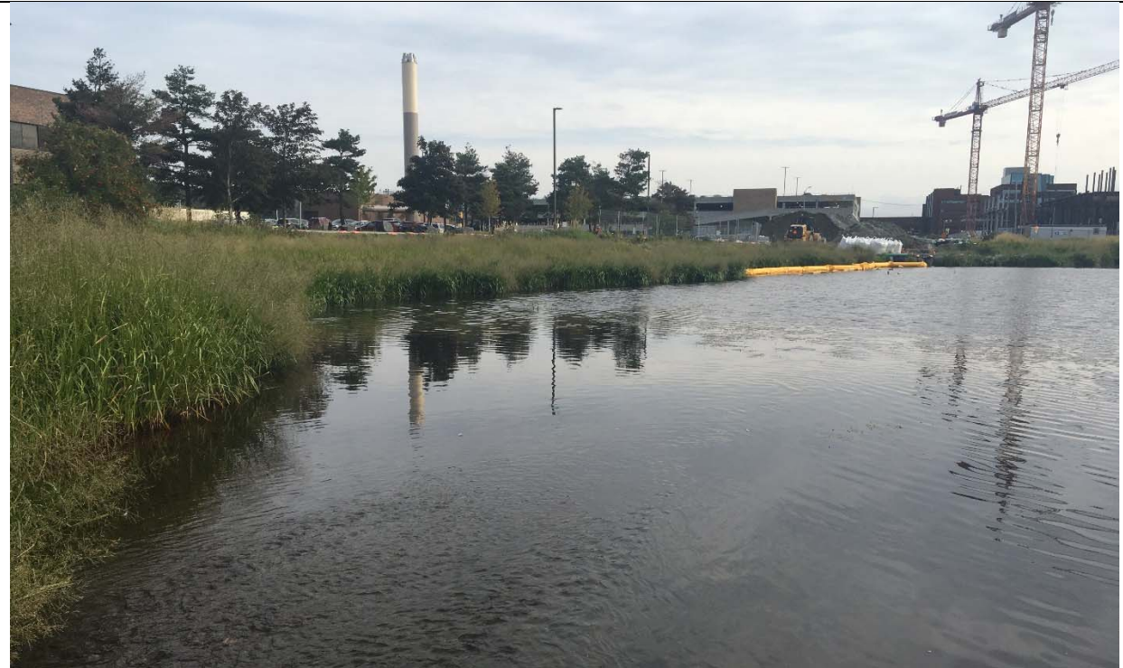
PHOTO 11: Poned area east of the HSC. Sediment control boom visible at site of retaining wall construction. Looking northeast.
