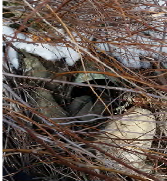
Figure 5: Existing Culvert Outlet
