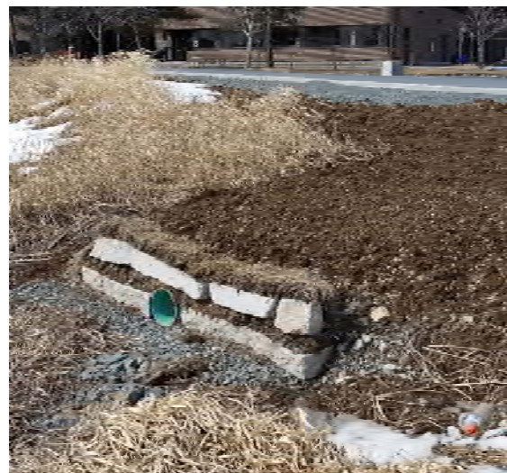
Figure 4: New Storm Sewer Outlet
