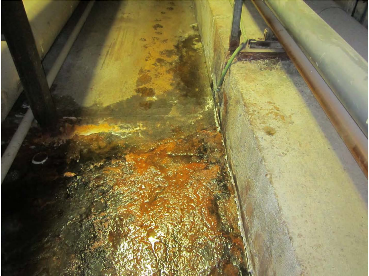
Photo 3 – Hose from sump pump
