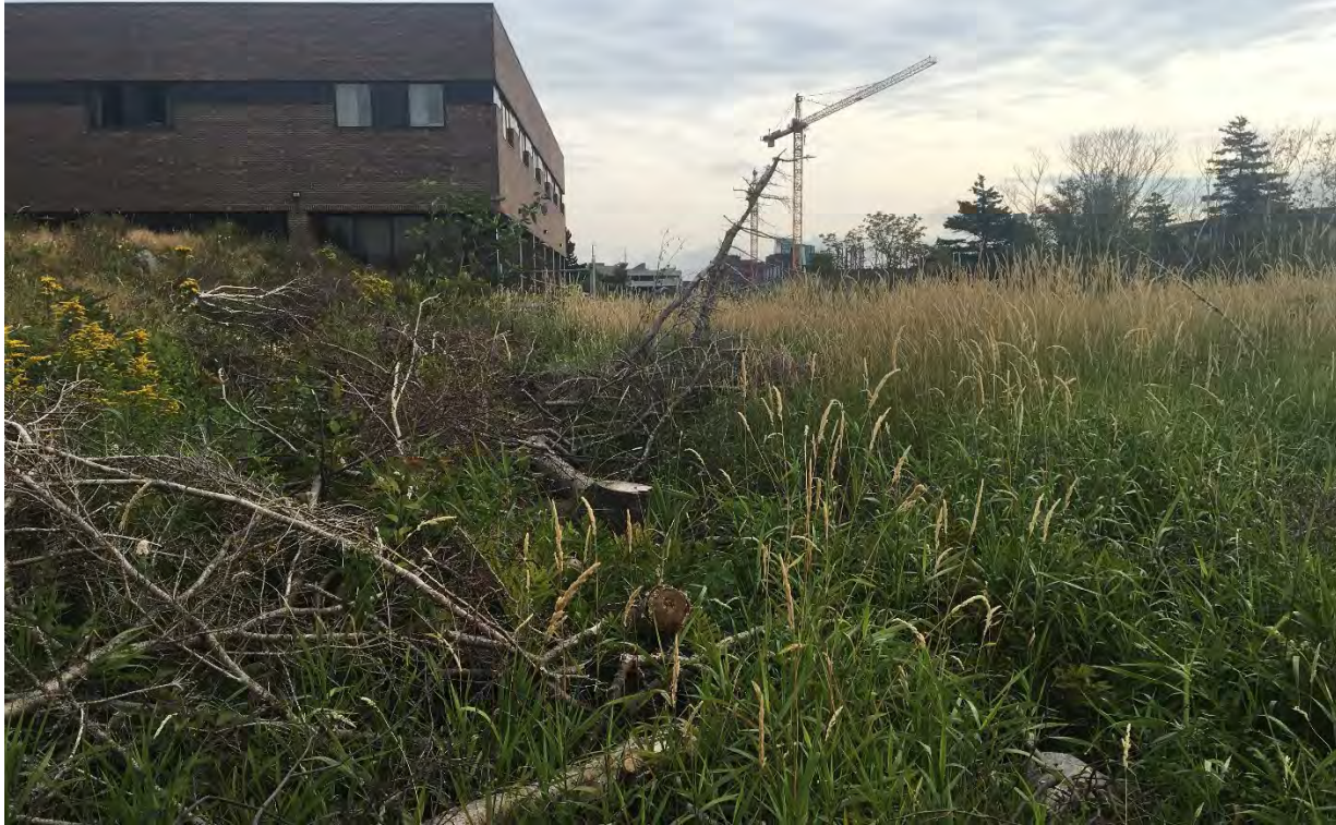
PHOTO 9: Some vegetation clearing has taken place at the periphery of the wetland and along the existing berm, in preparation for construction. Looking northeast.
