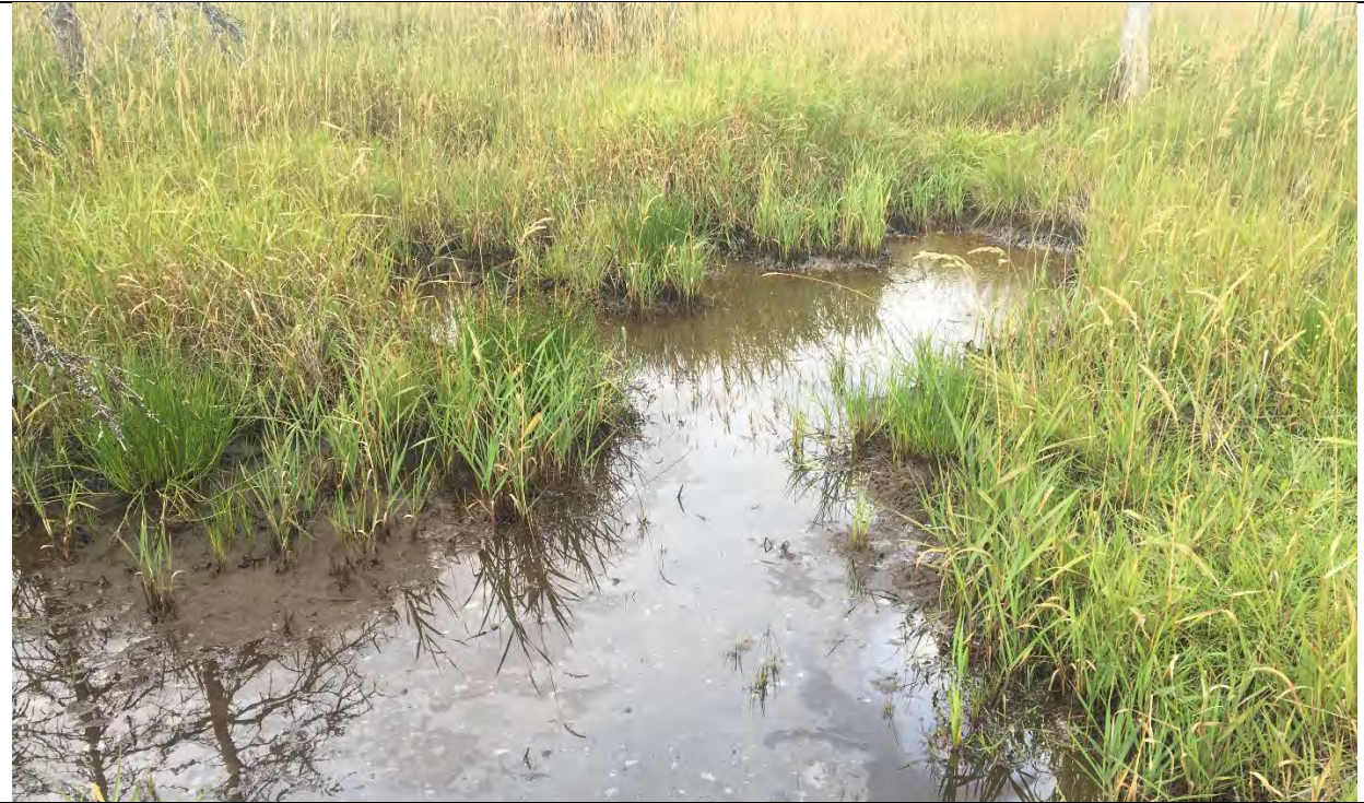
PHOTO 5: Typical conditions within pooled area down-gradient from stormwater outflow, adjacent to existing bank. Looking southwest.
