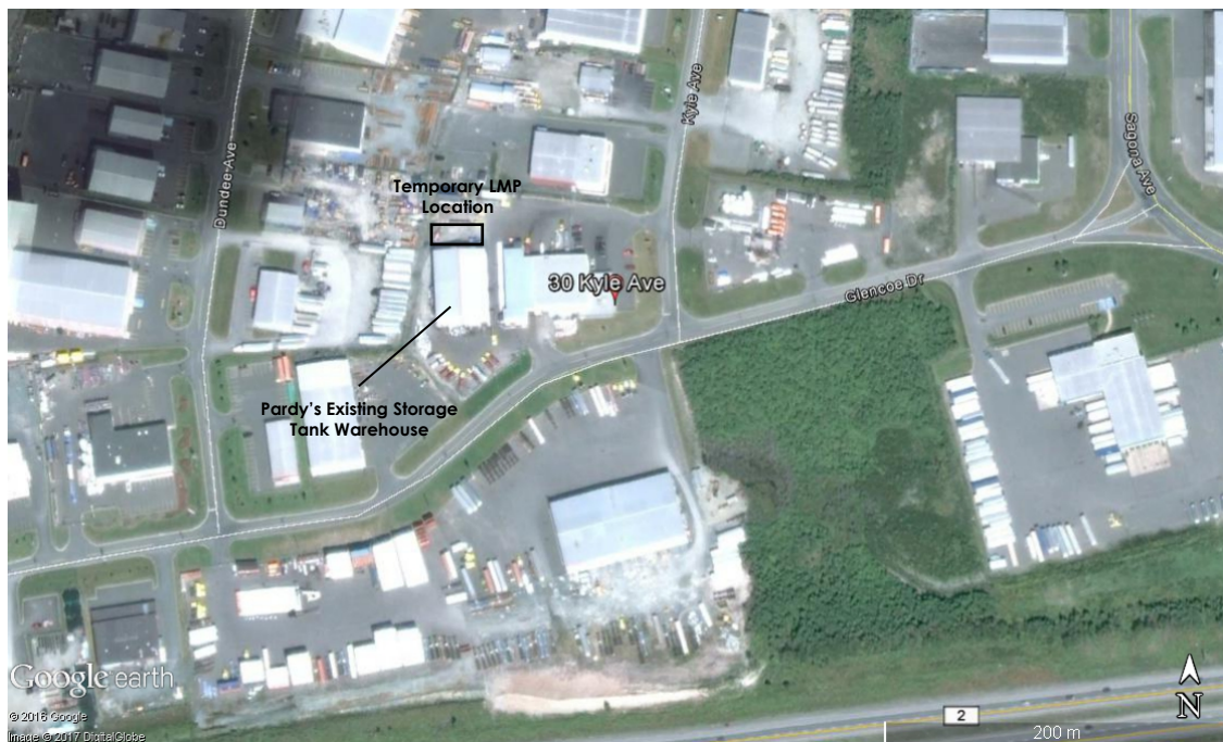
Figure 1 Temporary LMP Location
