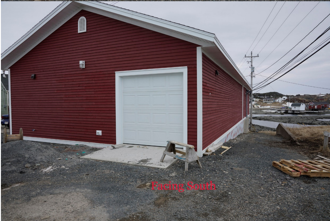
Facing South showing western side Concrete Property Divider
