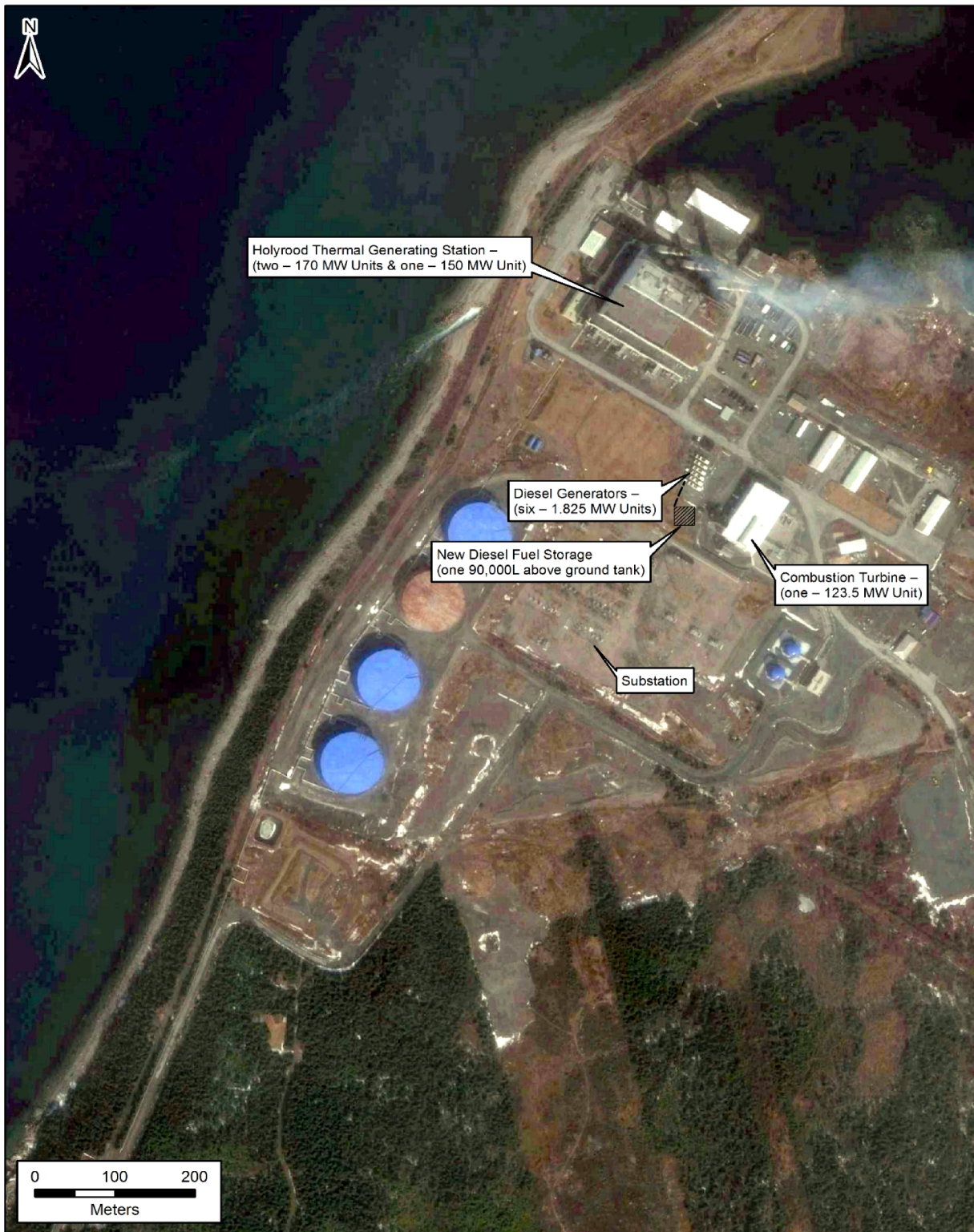
Figure 2.3 Location of the Diesel Generators on the Holyrood Thermal Generating Station Property
