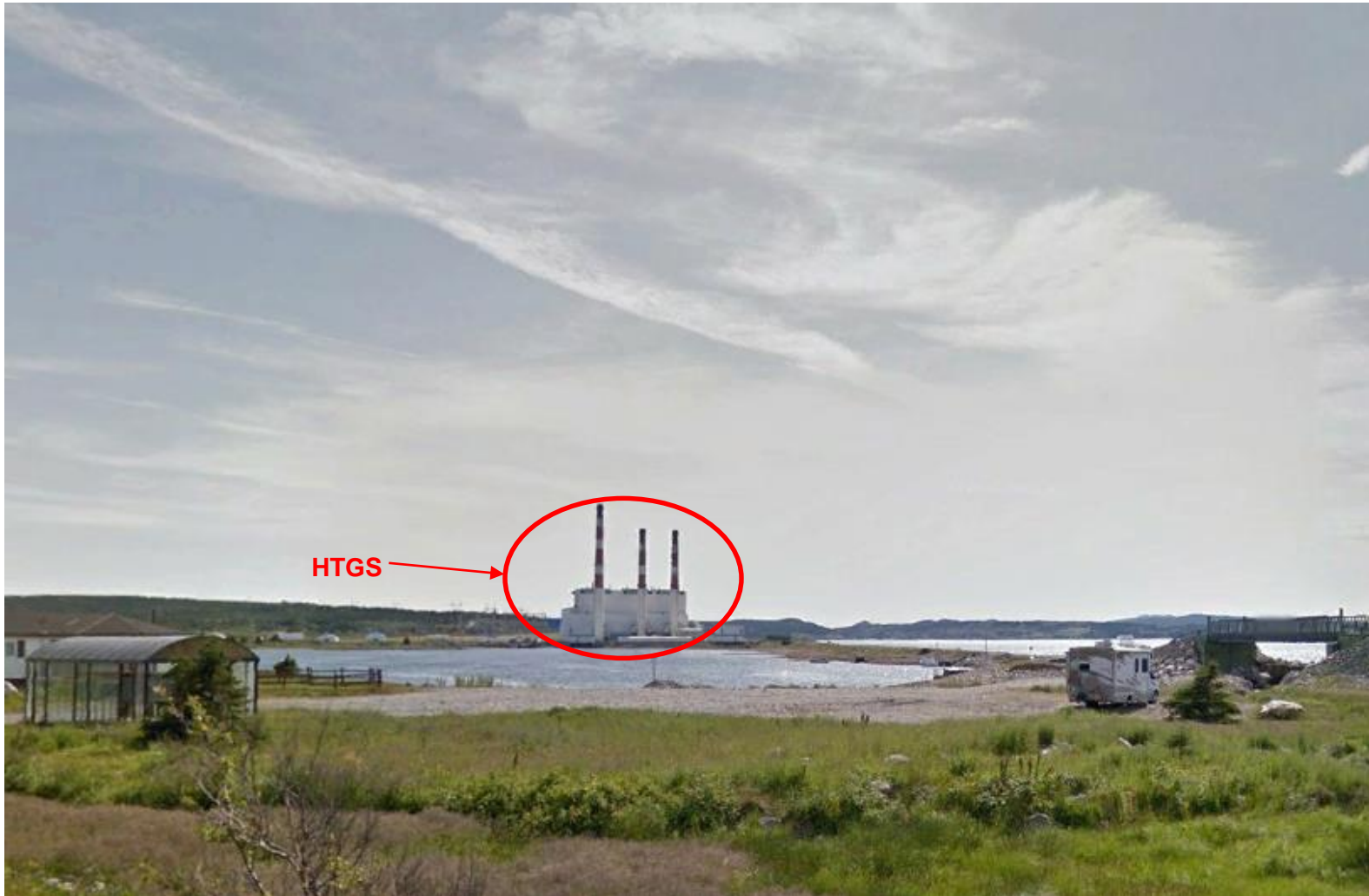
Figure 2: Site Photograph showing HTGS Units 1, 2 and 3
