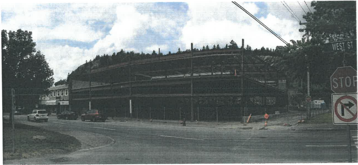
Image 3: The current state of the building after demolition is complete.
