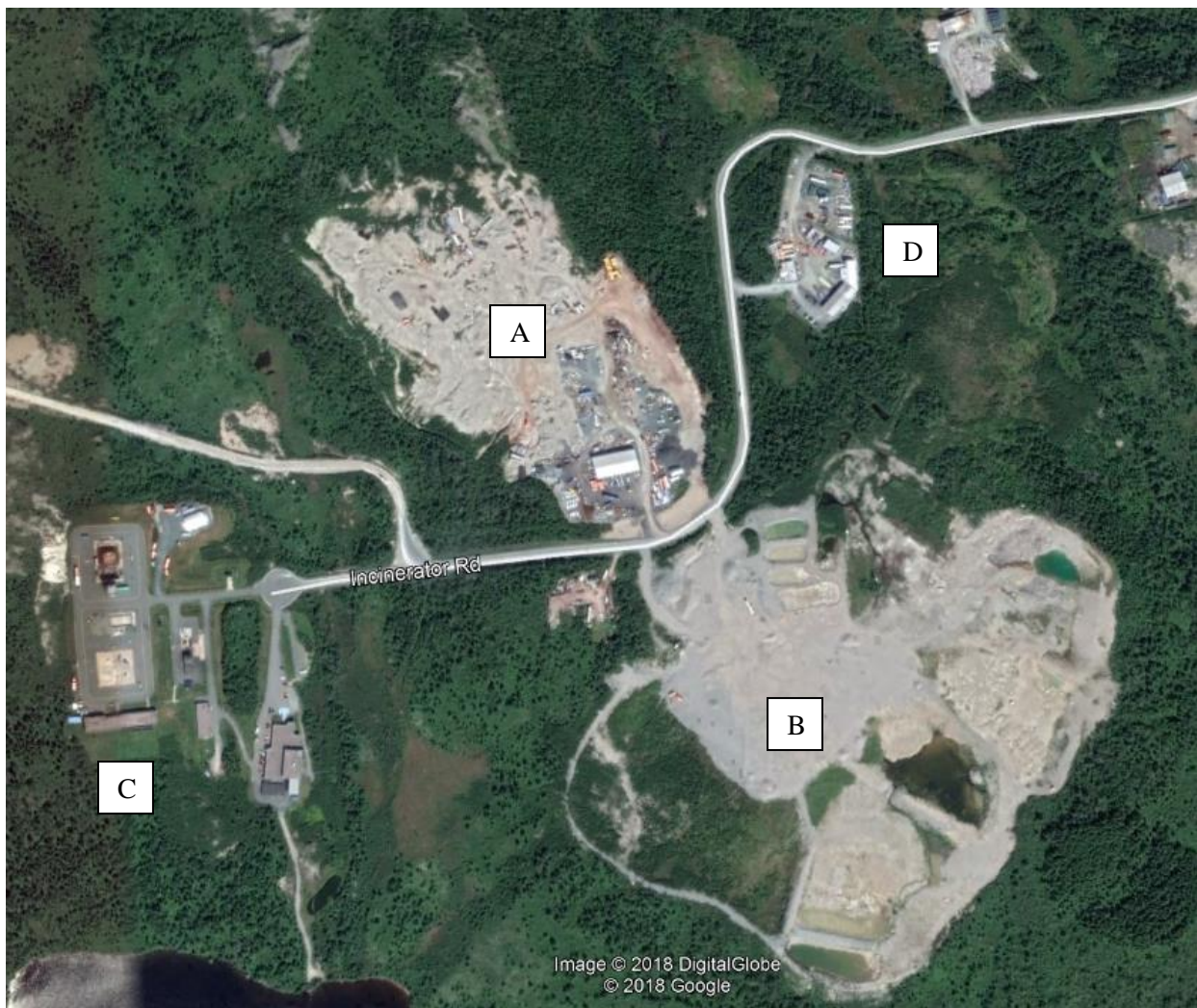
Figure 2: Google Earth Site Image
