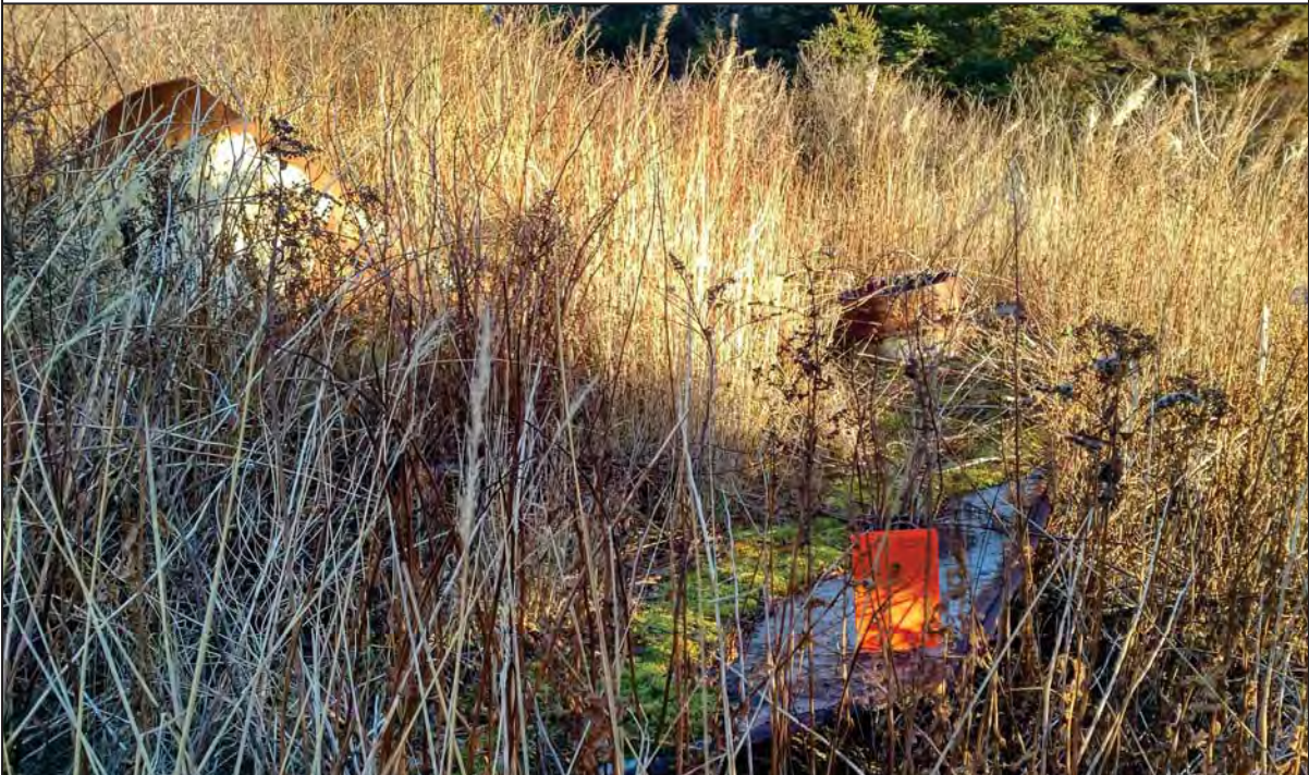
Figure 4 Large section of abandoned steel plate or a tank near the shoreline of the port of Stephenville.
