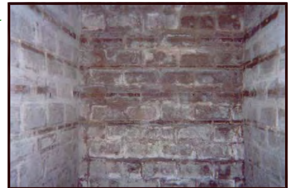
PHOTO 2: VIEW OF WALLS IN RECEIVER BUILDING FOLLOWING LEAD ABATEMENT.
