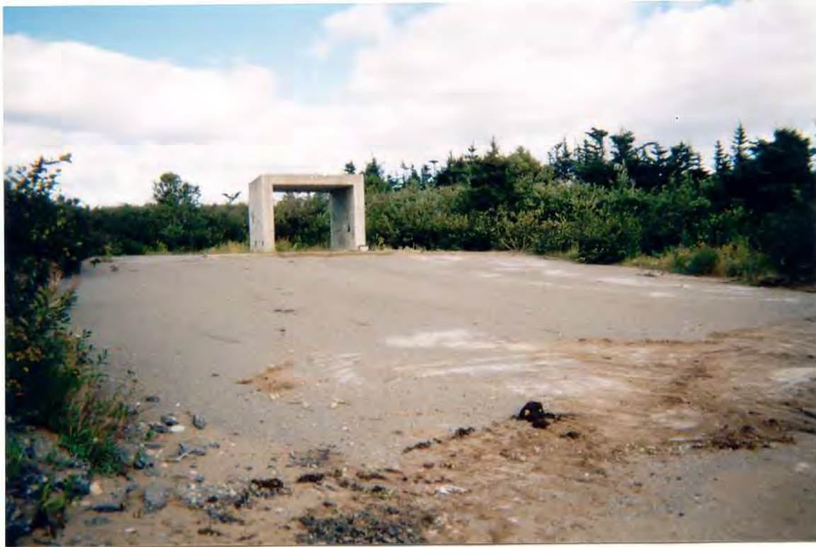
Photo G: View of EPU site facing northeast.
