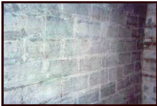
PHOTO 2: VIEW OF WALLS IN TRANSMITTER BUILDING FOLLOWING LEAD ABATEMENT
