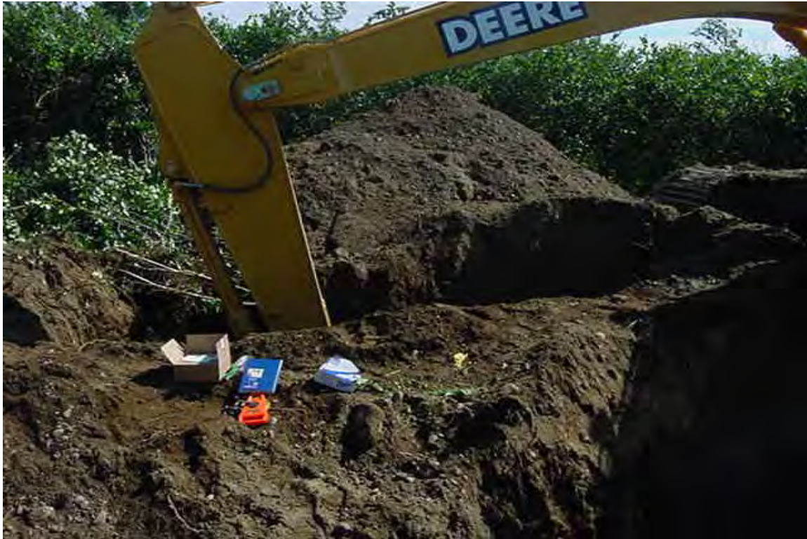
Photo A: Excavation of RX-TP1.
