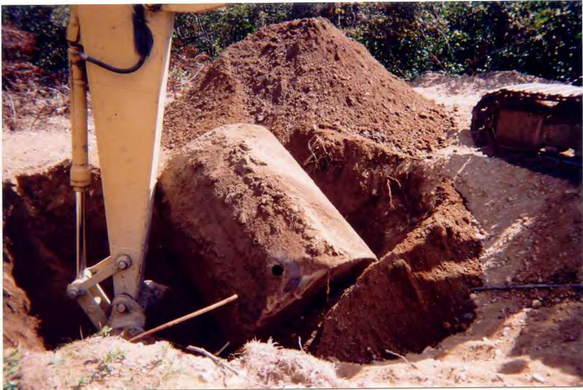
Photo F: UST adjacent to transmitter site after removal.
