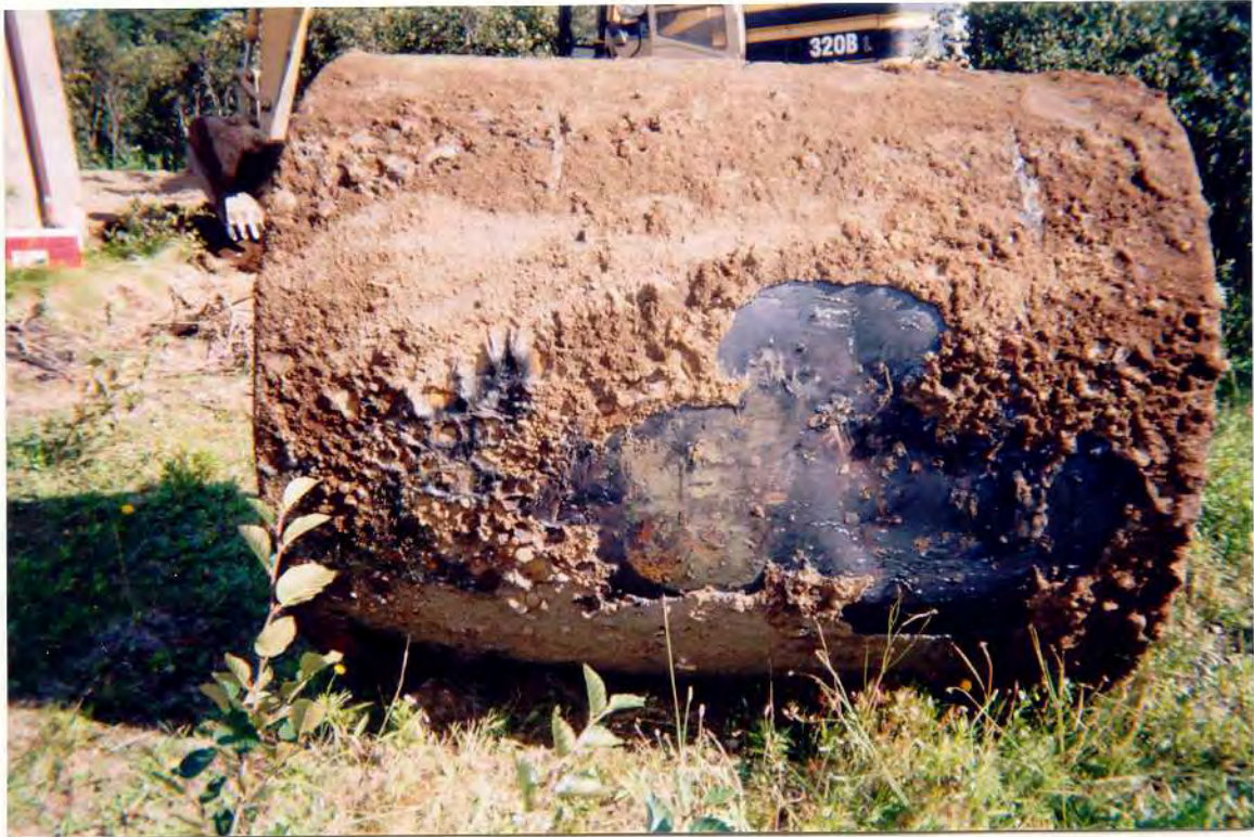
Photo E: UST adjacent to receiver site after removal.
