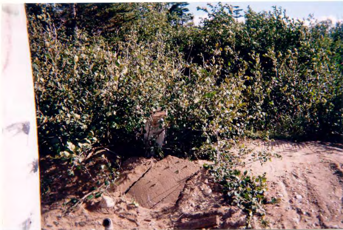
Photo H: View of AST cradle location at EPU site.
