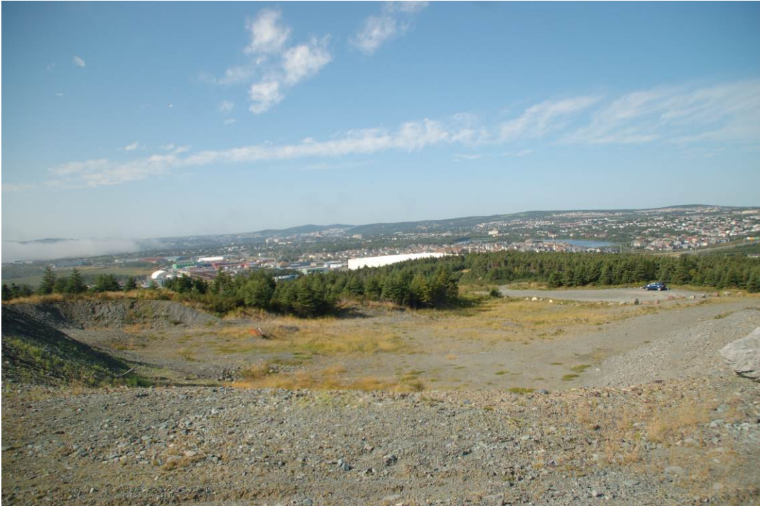
Cleared land at front of site.
