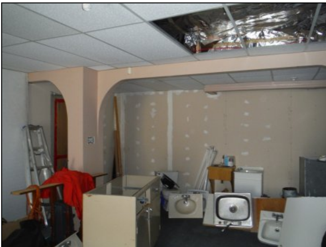
Storage of miscellaneous materials on the first floor of the site building
