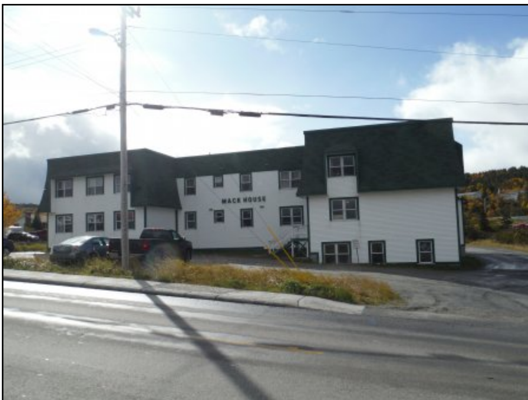
Neighbouring property (Mack House) to the south, across West Street, looking south
