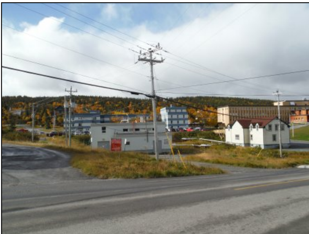
Neighbouring properties (Boiler Building and Boys and Girls Club) to the southwest, looking southwest
