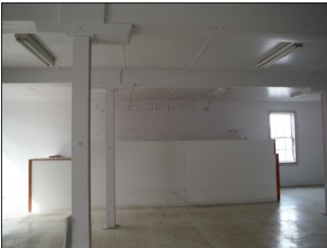
Building interior in the 1935 portion of the site building
