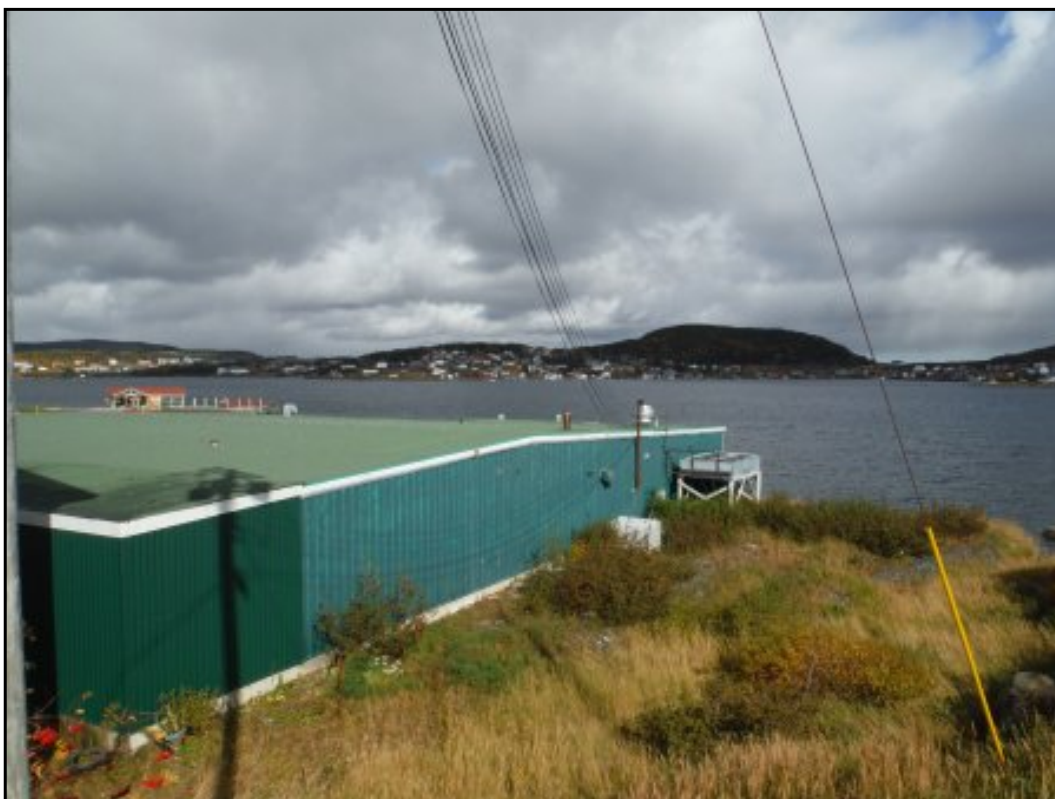
Down-gradient adjoining property (Co-Op) with two exterior ASTs on the southeast side of the building, looking north
