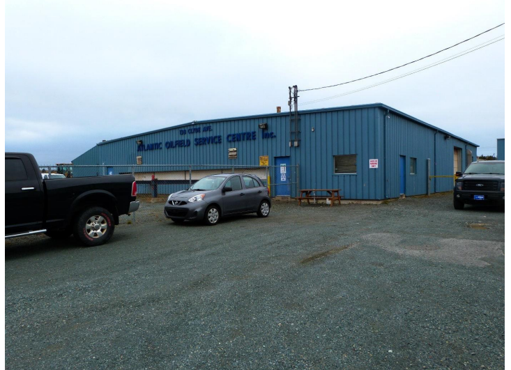
Existing building and Fence
