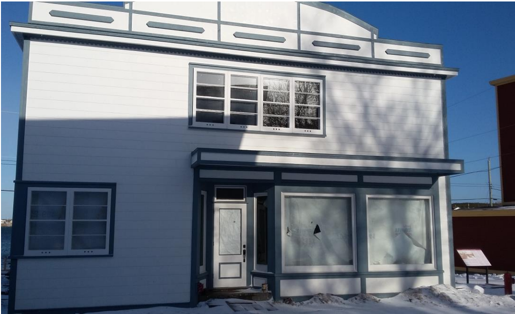
Figure 3: Street - level view of the main entrance at the Union Electric building at 49 – 53 Main Rd, Port Union, NL.
