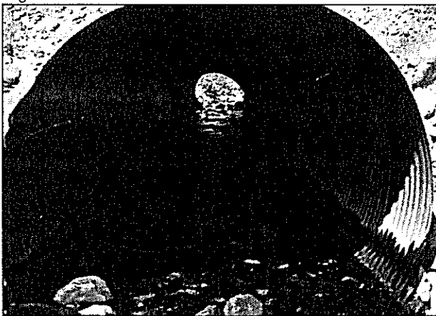
Figure 3. Countersunk Culvert
