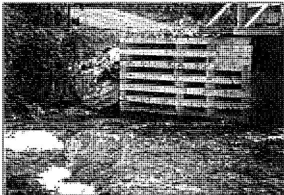
Timber crib construction: untreated/pressure treated wood.
