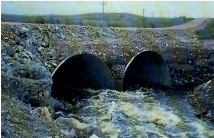
(a) Bottomless arch installation.
