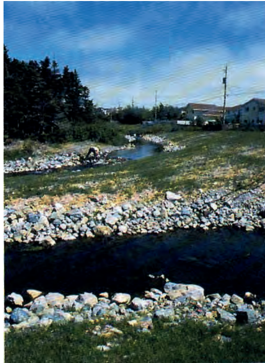
Figure 4.14 Rock riprap prevents erosion.
