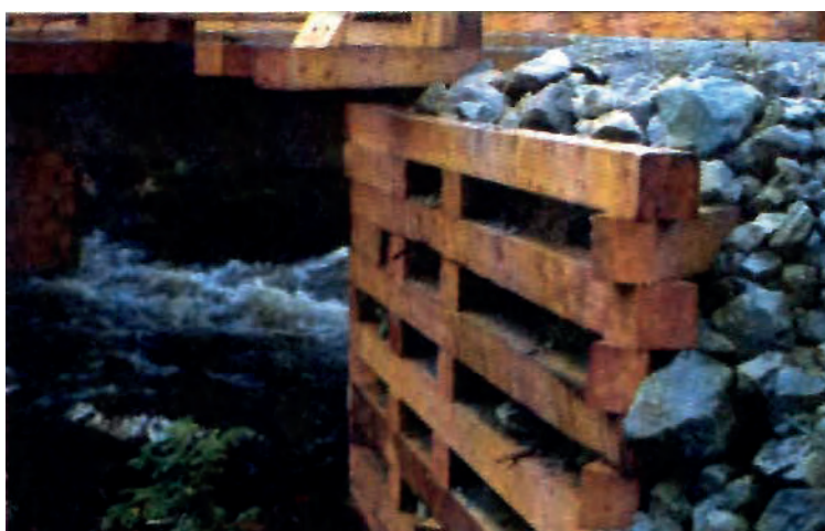
Figure 4.15 Infill materials for timber cribs should be blocky, angular and free of fines or sediment.
