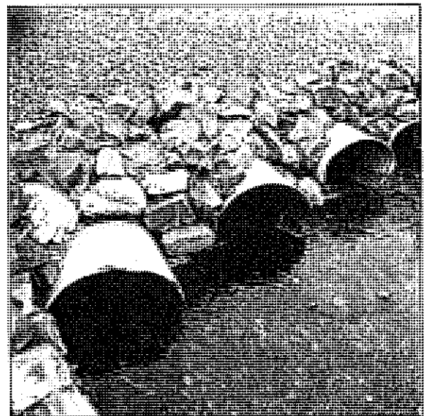
Stabilization of culvert outlets - rip rap.
