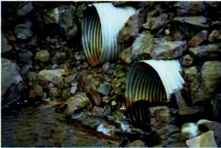
Figure 4.22 Multiple Culvert Installation
