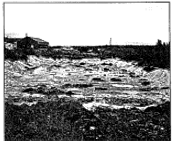
Settling basin lined with plastic.
