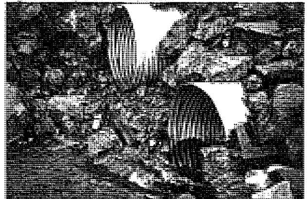
Figure 4. Multiple Culvert Installation
