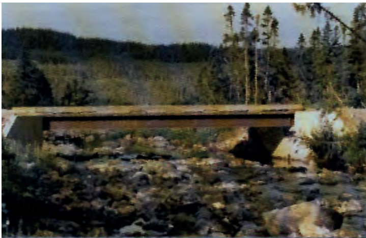
(b) Permanent bridge.
