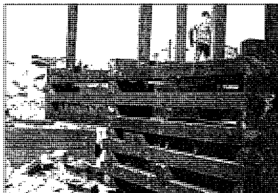
Timber crib construction for marine environment.
