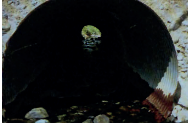
Figure 4.21 Countersunk Culvert.
