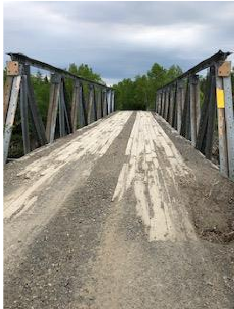
Photo 3 Victoria River Bridge
