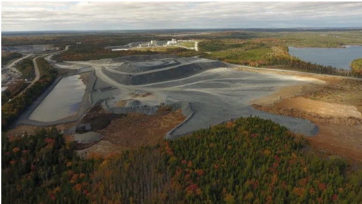
Figure 2-10 Typical Sedimentation Pond
