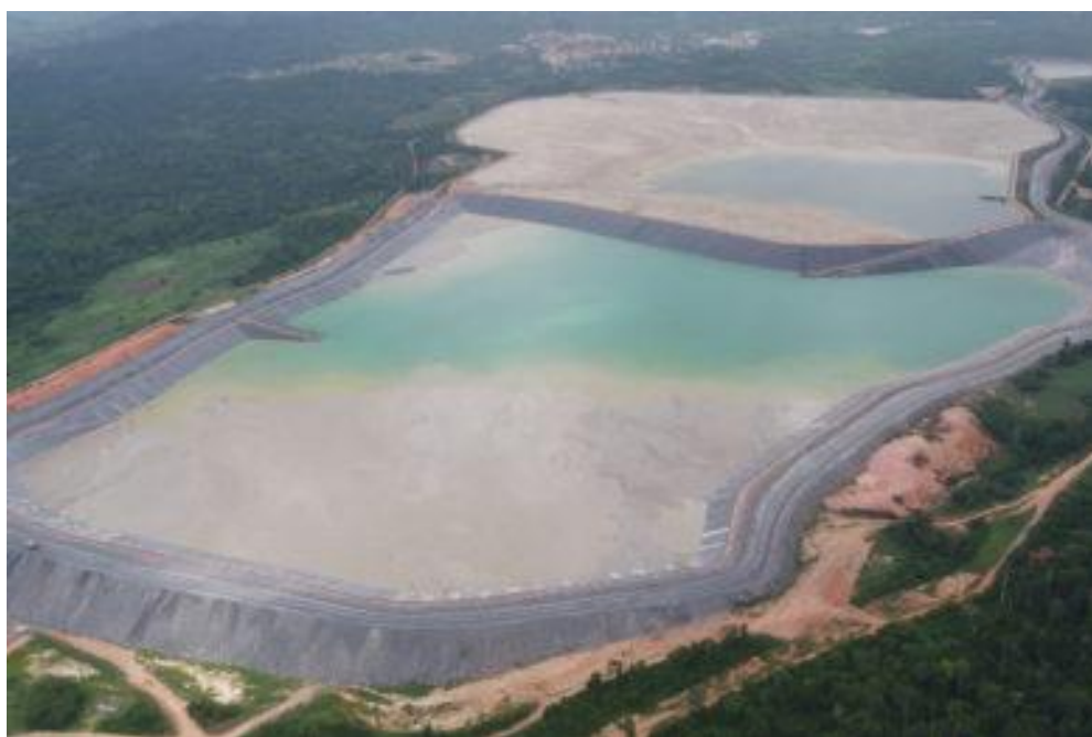
Figure 2-8 Typical Tailings Management Facility
