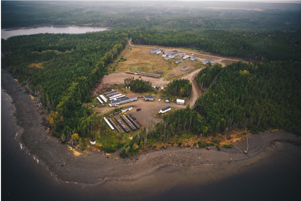
Photo 1 View North, Existing, Permitted Marathon Exploration Camp
