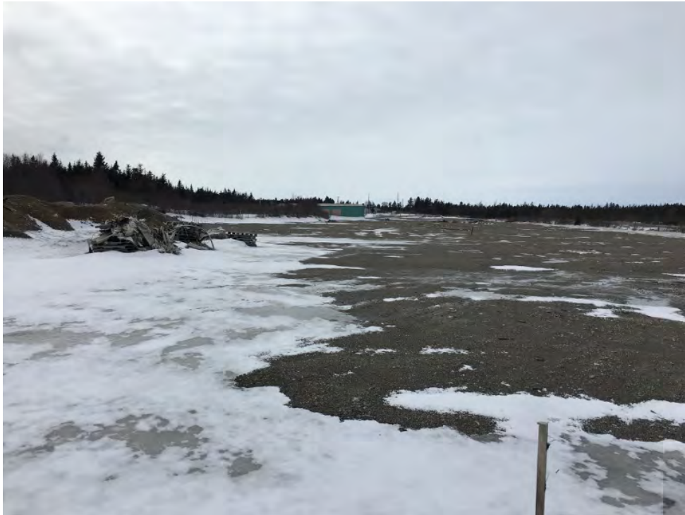
Photo 4 – View, looking west, toward Warehouse (former Repair Shop) and across former laydown yard with miscellaneous debris at left of photograph (provided by Back Home Grow).
