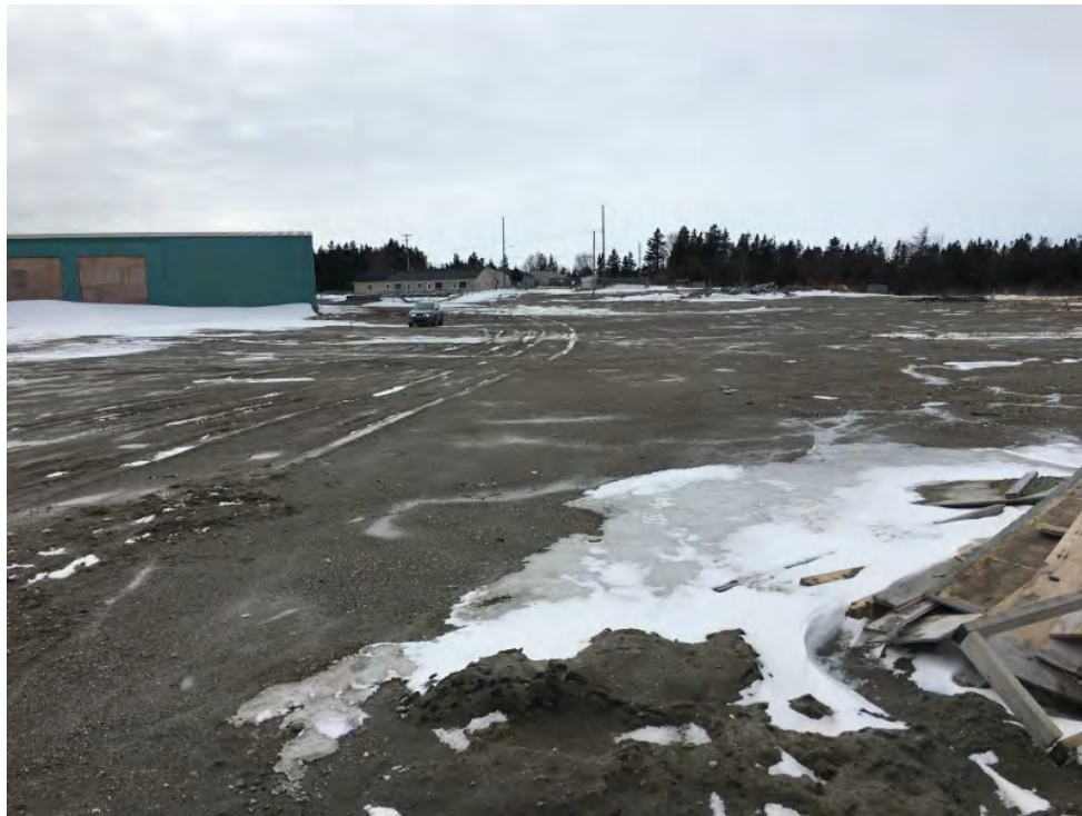
Photo 5 – View, looking southwest, toward Warehouse (former Repair Shop) and Main Office (provided by Back Home Grow).
