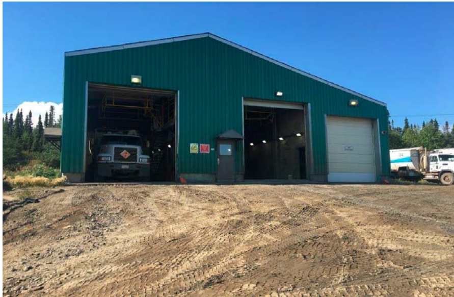
Figure 6 Existing Wash Bay
