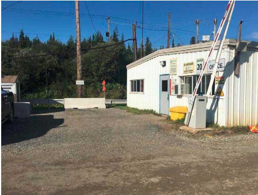
Figure 5 Existing Administrative Building
