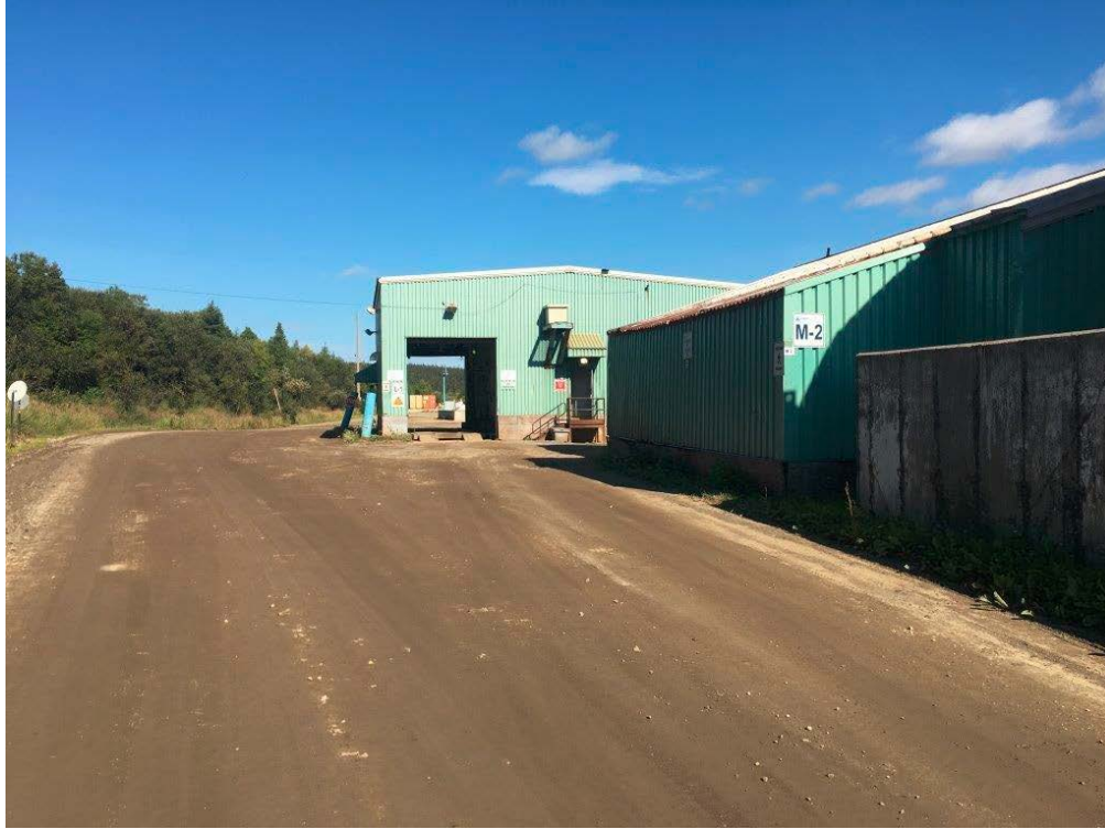
Figure 8 Existing Production Building
