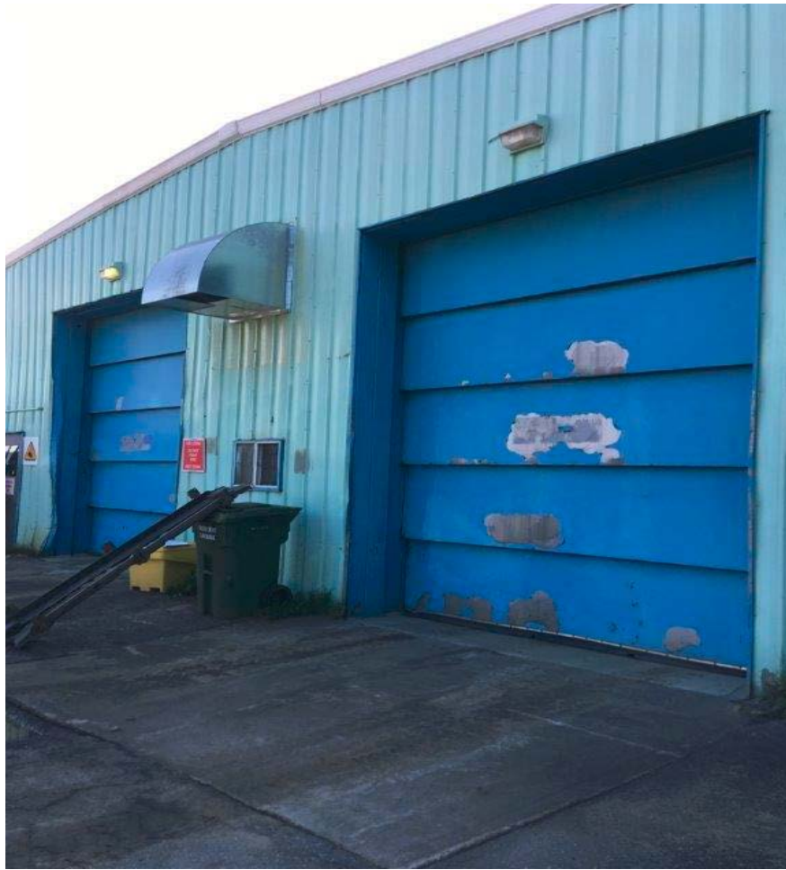
Figure 7 Existing Maintenance Garage
