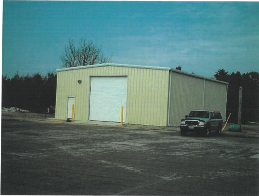
Figure 3: Site Building Example
