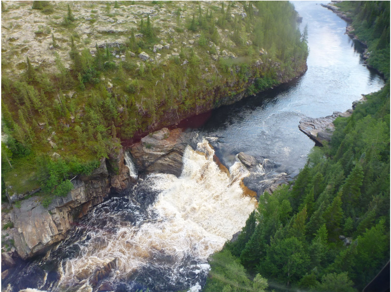
Figure 3-1 St. Lewis River Falls at Km 28 View from North side showing the rock fracture run-around along the South side, on the left
