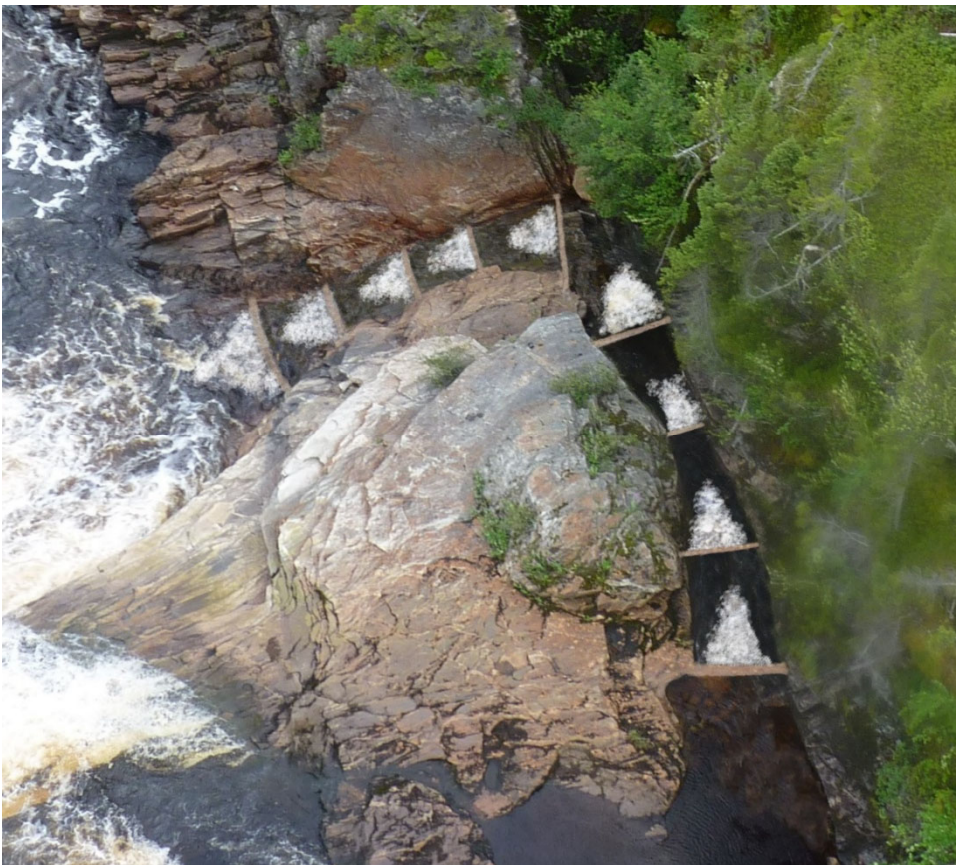
Figure 4-1 Fish passage concept with concrete baffles creating pools in the run-around flow pathway occurring at the falls located at km 28
