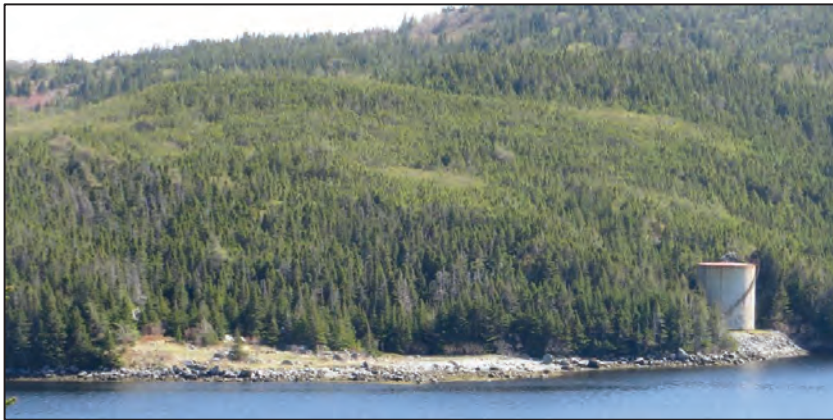
Looking south from the road to Port Kirwan towards the clearing at Lawes Point (centre, and to left), showing a fuel storage tank (RCF.2304).
