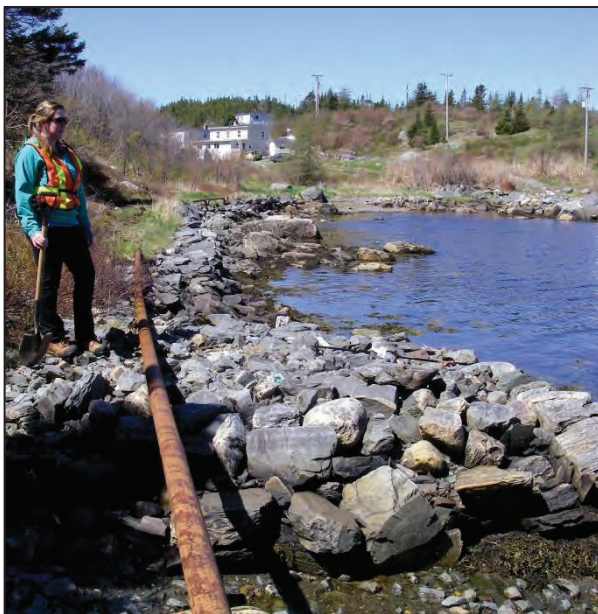
Ballast bed (wpt "Ballst") and quay/roadbed, looking towards Brophys Brook (BTF.3617).
