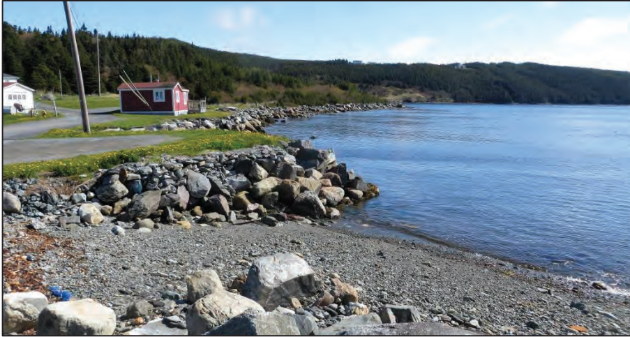
The west side of Rumley Cove, looking north along a transformed shoreline, towards Ships Head (RCF.2241).
