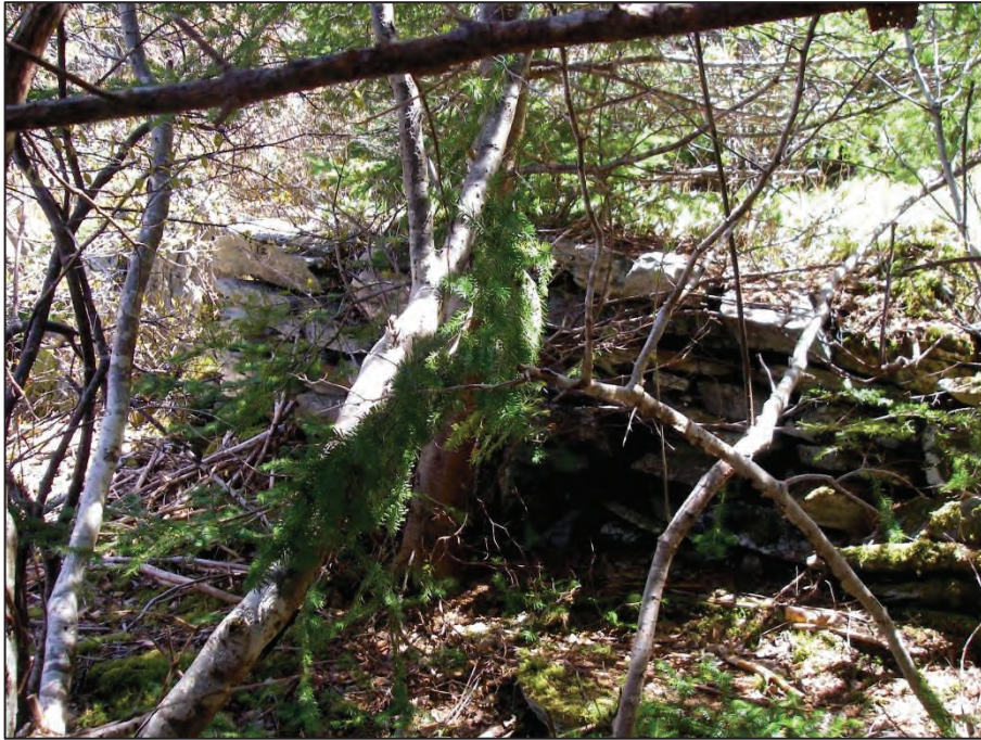
Roadbed at Steel Point (BTF.3674).
