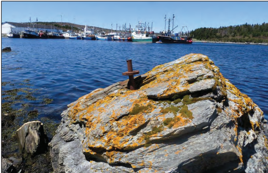
Warping pin set in a rock on the east side of Rumley Cove (RCF.2265).
