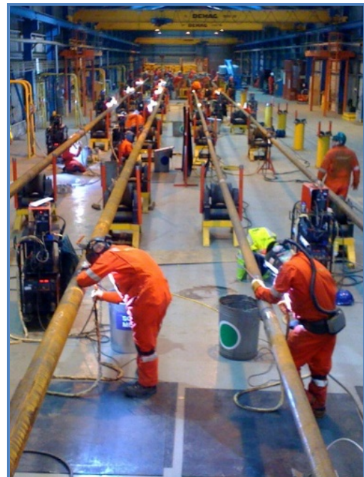
View Inside Fabrication Building
