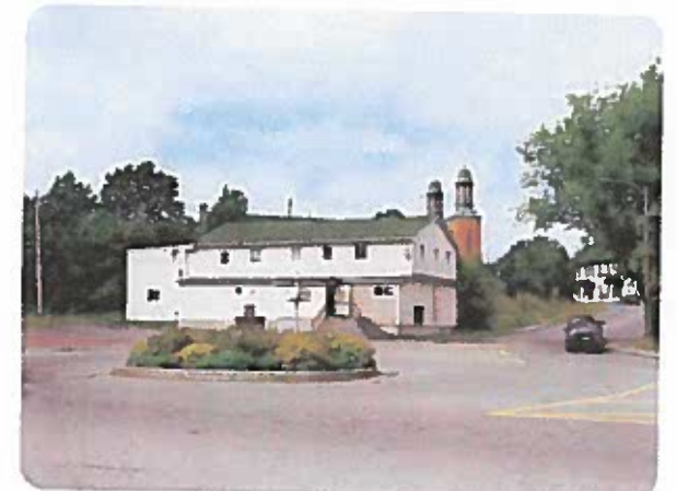
View of roundabout in Grand Falls
