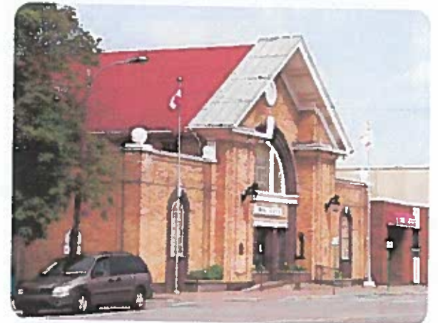
Town of Grand Falls-Windsor Town Hall
