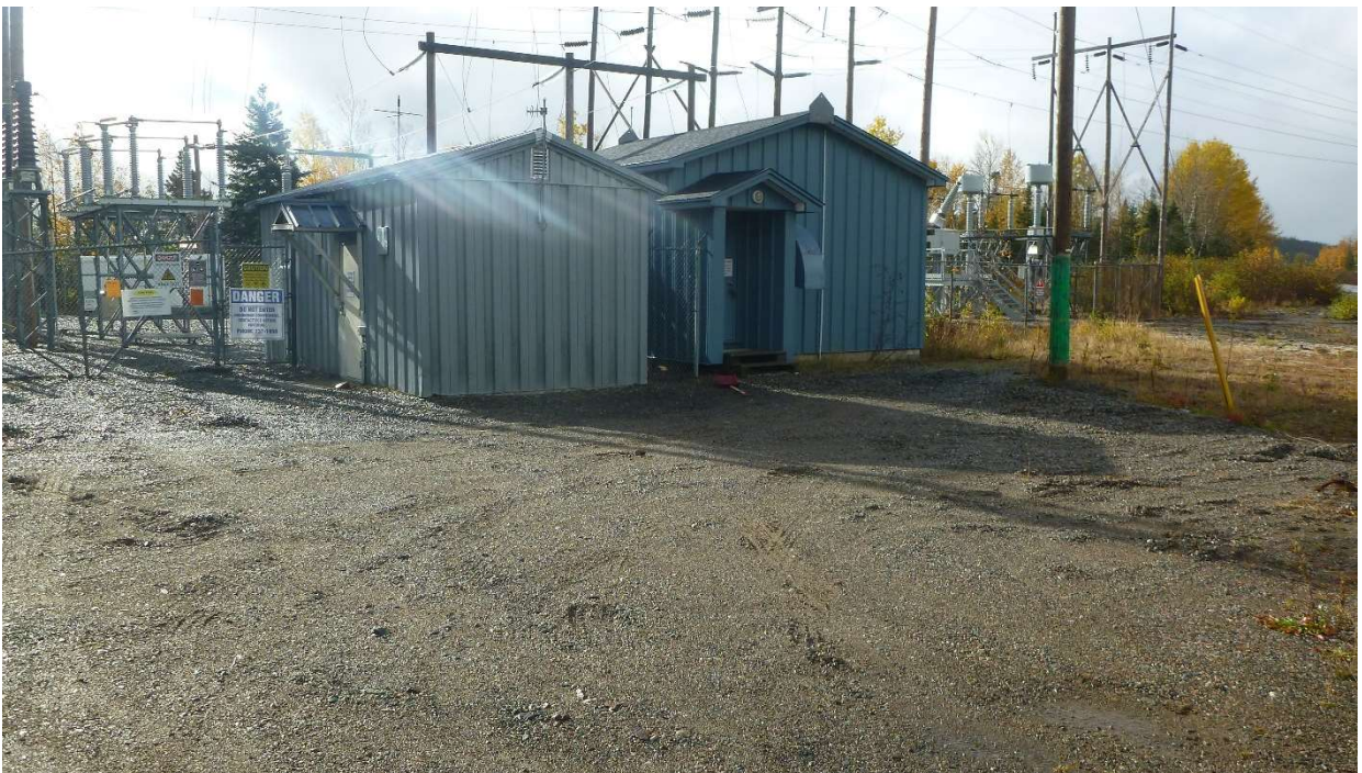
Photo 12: View of Terminal Station Buildings near Route 392.
