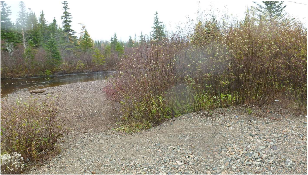
Photo 5: Heavy brush and sediment on overbanks downstream of Route 392 culverts.
