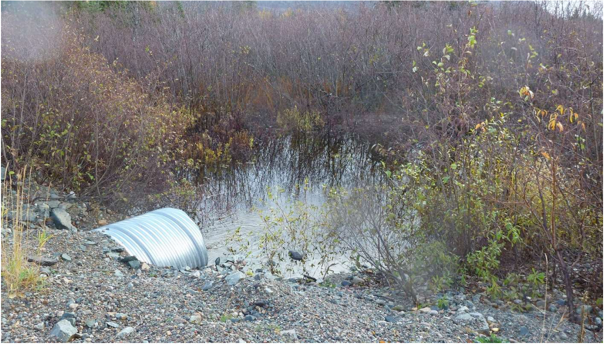
Photo 9: Downstream of cross culvert at Route 392.
