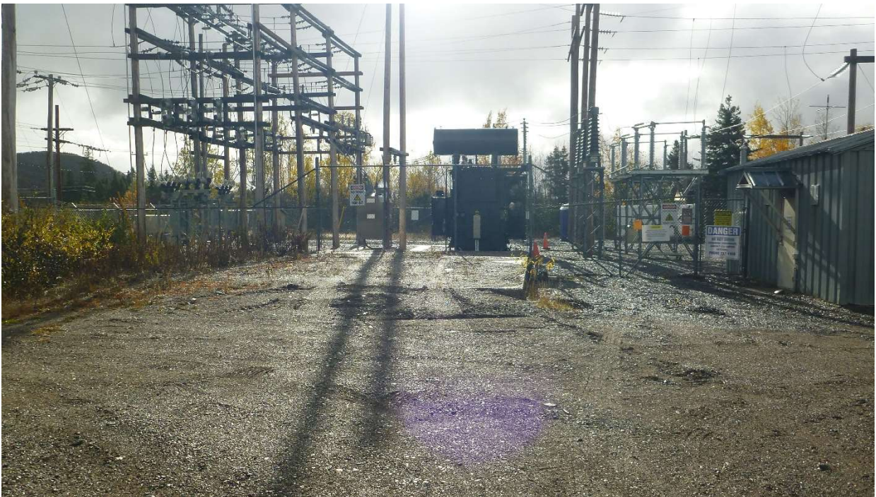
Photo 14: Terminal Station Building and concrete pad looking south.
