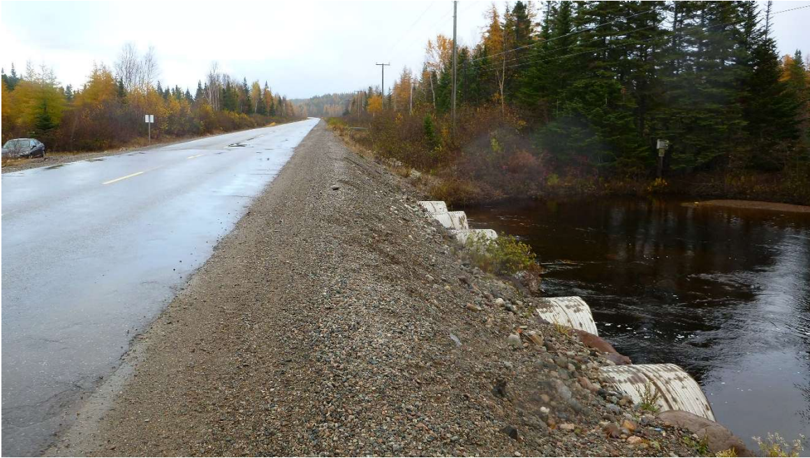
Photo 2: Downstream culvert structure at Route 392 looking northeast.
