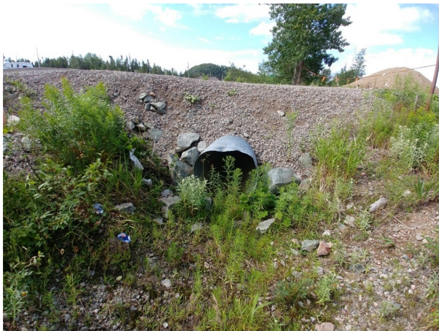
Figure 19: Option 2 Site Visit Observation 2e – 900mm Accessway Culvert on Route 392
