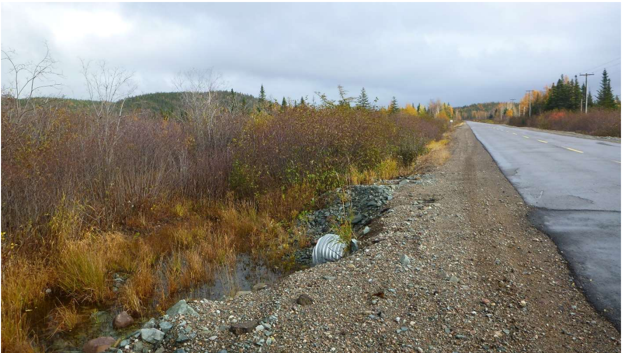
Photo 8: Upstream of cross culvert at Route 392 looking northeast.
