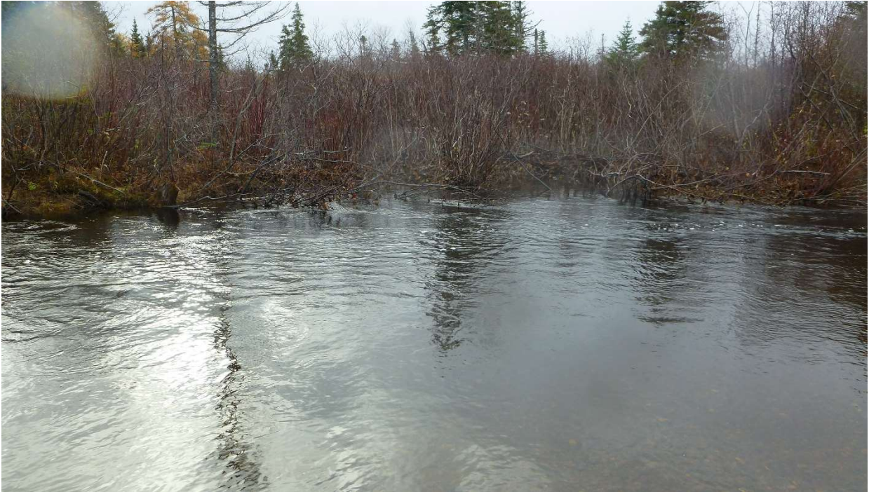
Photo 23: Flow passing through woody debris in Davis Brook Channel Near Route 392.
