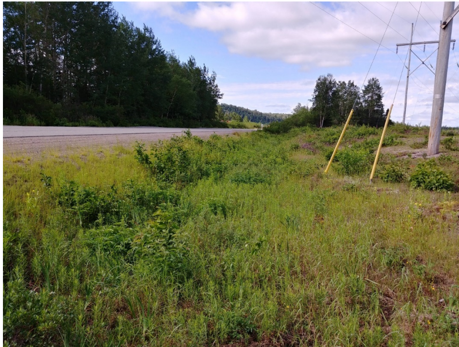
Figure 22: Option 2 Site Visit Observation 4 – Transmission Line Guy Wires Near Existing Ditch
