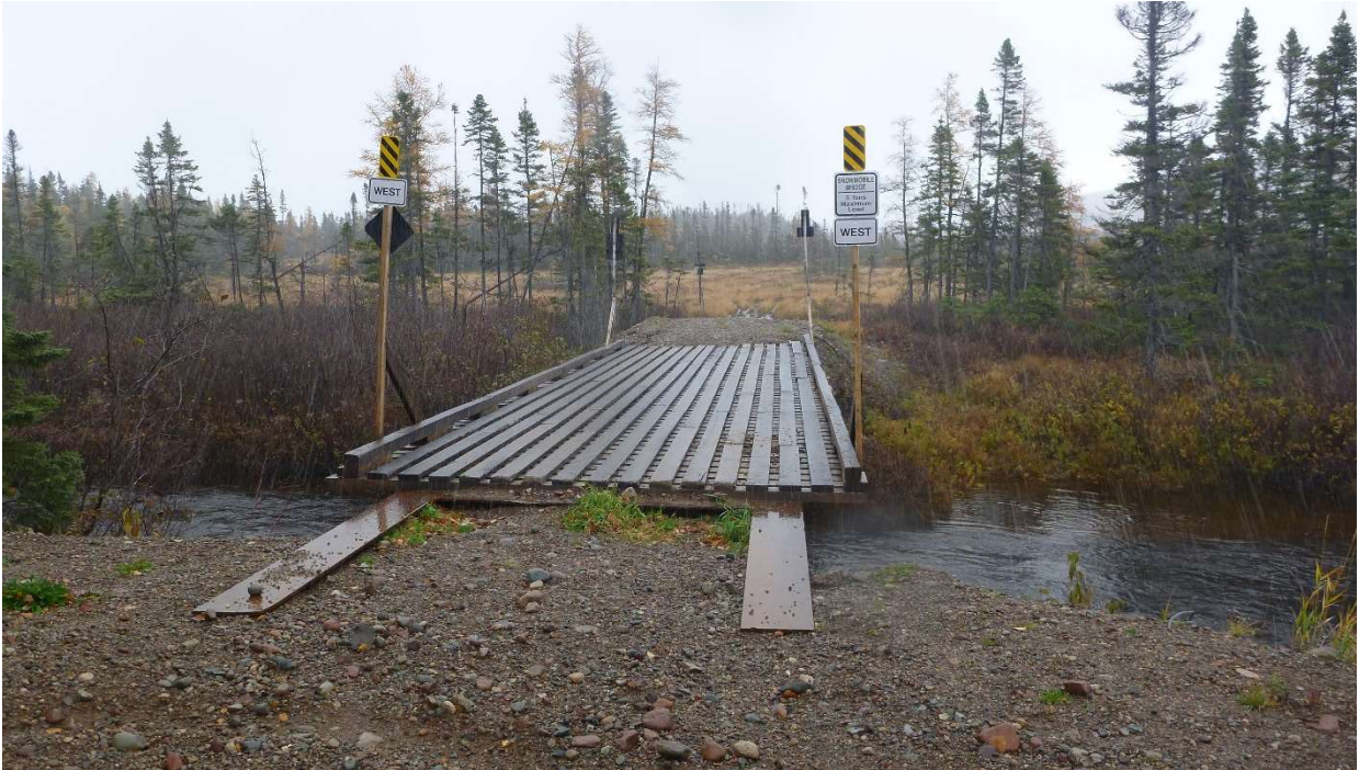
Photo 21: T'Railway bridge across Davis Brook.
