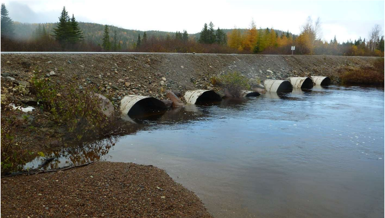
Photo 7: Downstream culvert structure at Route 392 looking north.
