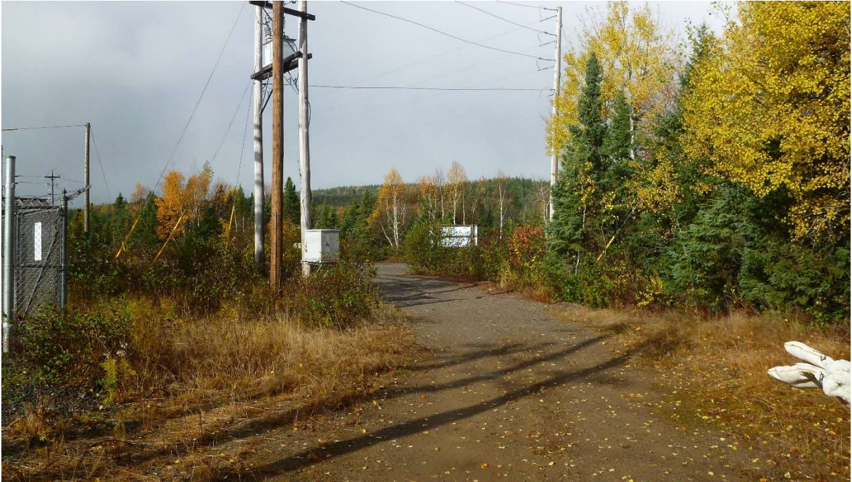
Photo 15: Terminal station access road from Route 392.
