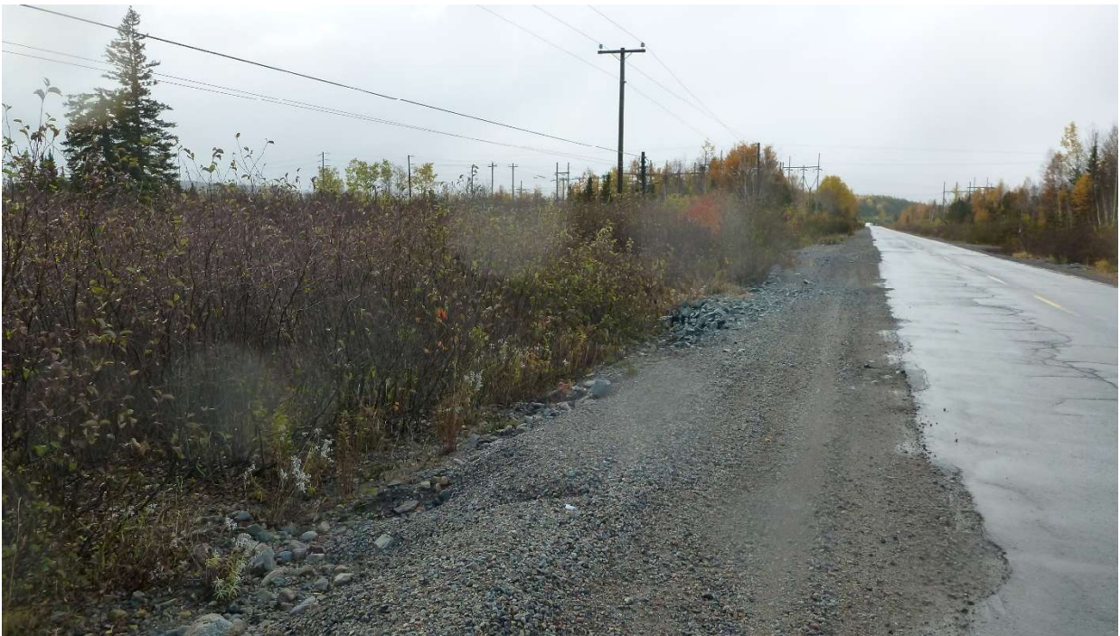
Photo 24: Route 392 looking southwest.
