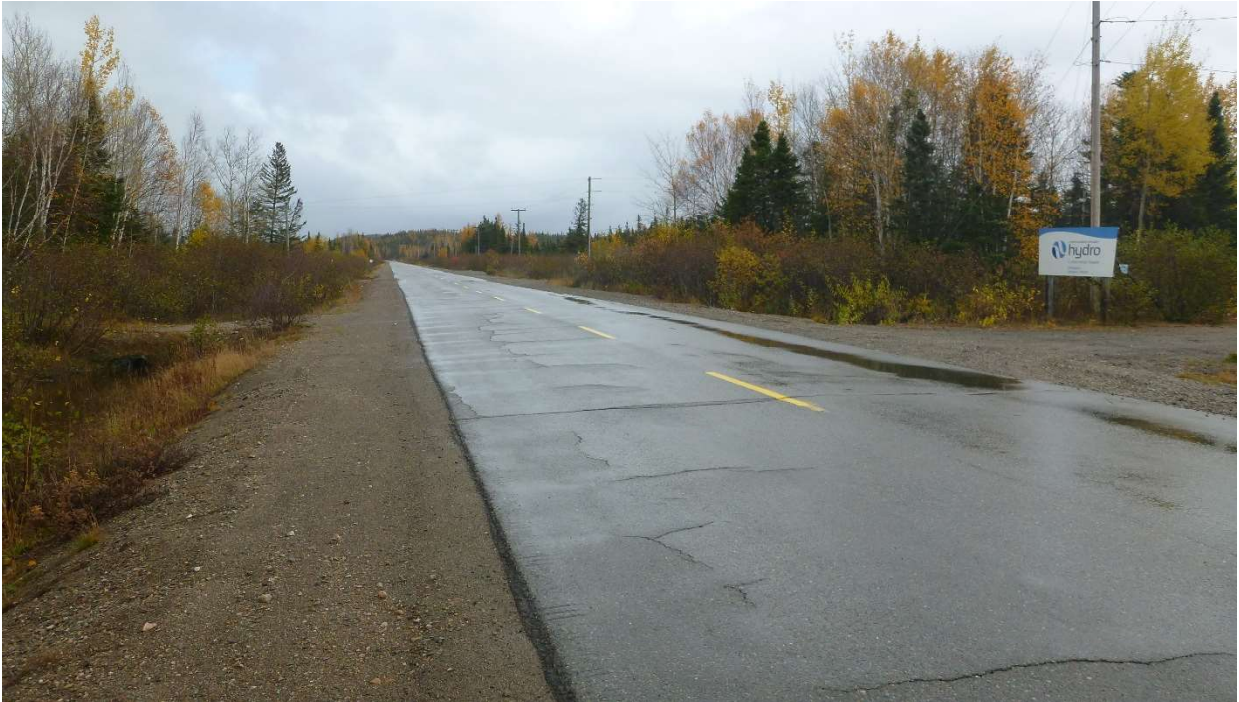
Photo 13: Entrance to Terminal Station from Route 392.
