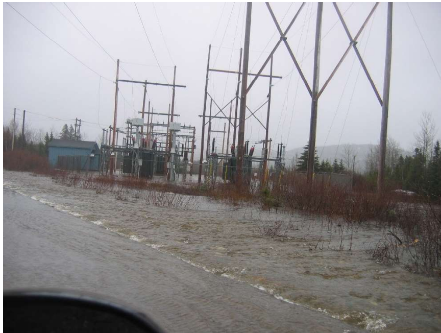
Figure 4 Flooding at Terminal Station (April 18, 2006) – Photo 1
