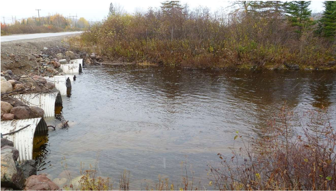
Photo 1: Upstream culvert structure at Route 392 looking southwest.
