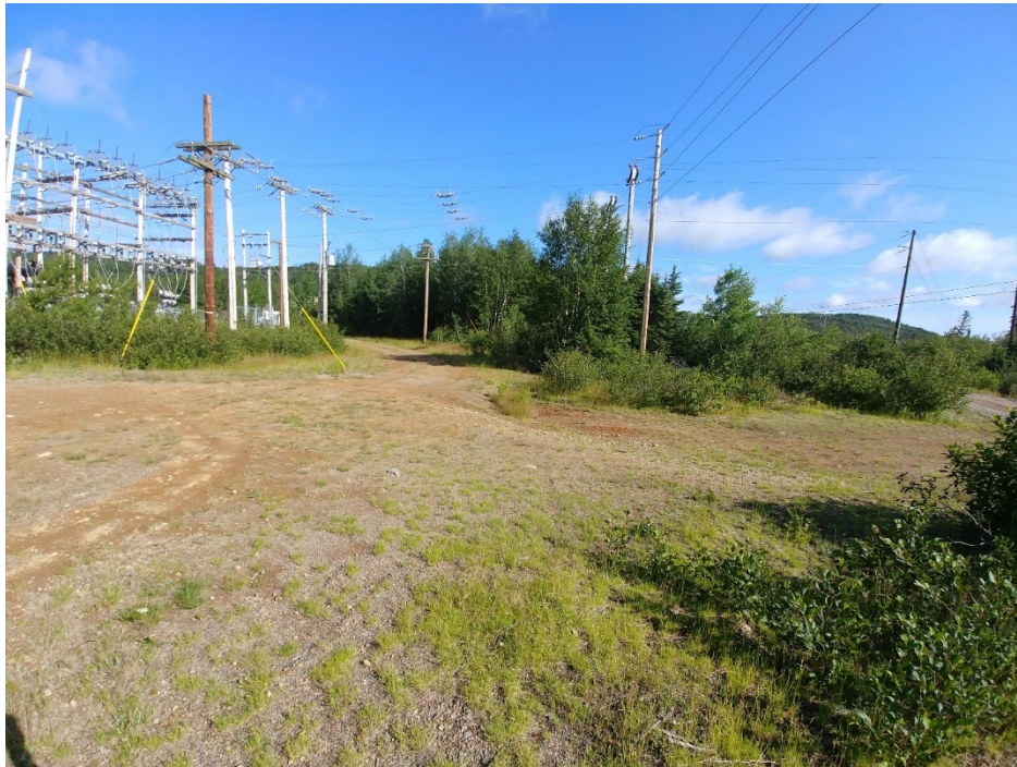
Figure 11: Option 1 Site Visit Observation 7 – Existing Pole Infrastructure Near Terminal Station
