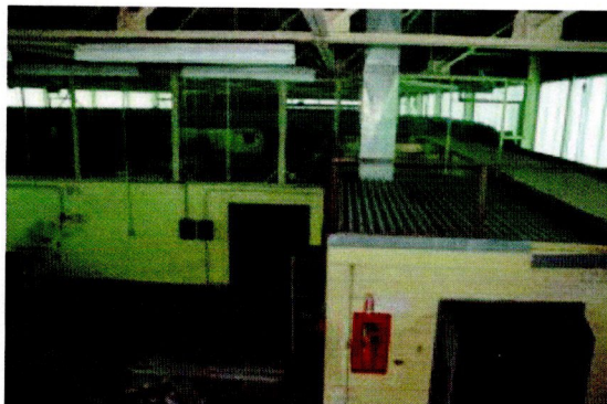
Outfit and Stores Building Interior
