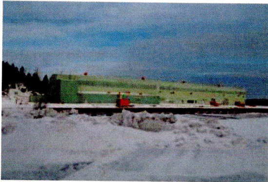
Outfit and Stores Building Exterior
