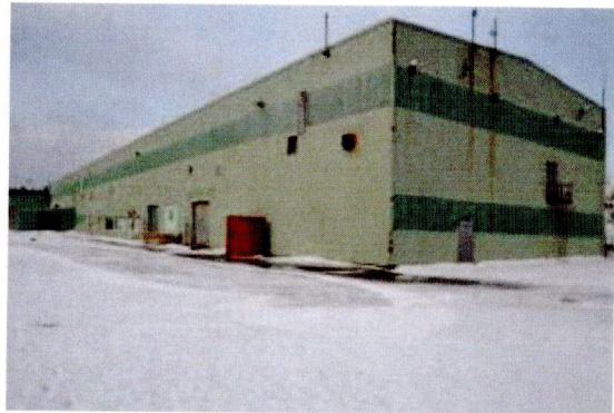
Outfit and Stores Building Exterior
