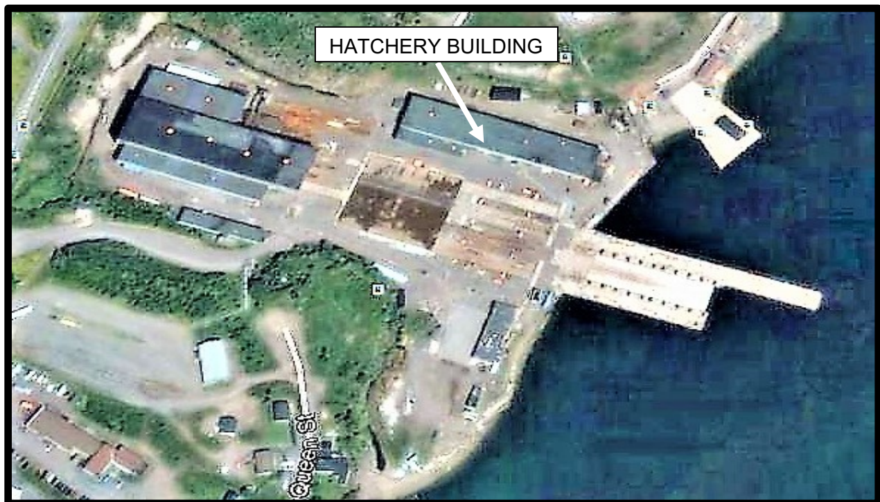
Figure 3: Marbase Cleanerfish Hatchery- Location in Marbase Service Hub
