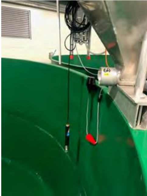
Figure 4.16: Optical oxygen tank probe sensor(s) and tank water level probe
