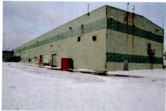
Outfit and Stores Building Exterior
