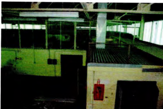
Outfit and Stores Building Interior
