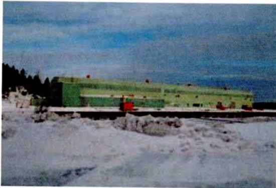
Outfit and Stores Building Exterior
