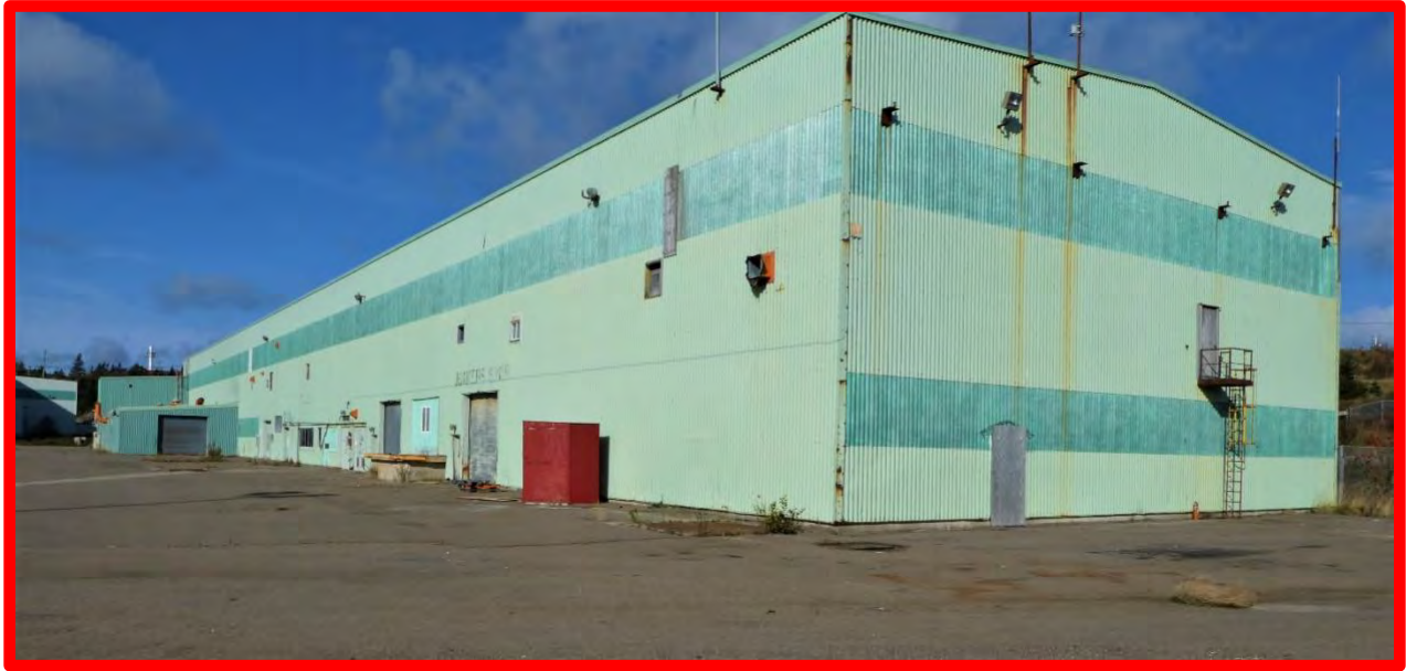
Hatchery Building looking West (Nov. 2020)
