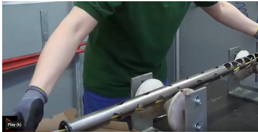
Figure 15. Installation of detonating cord
