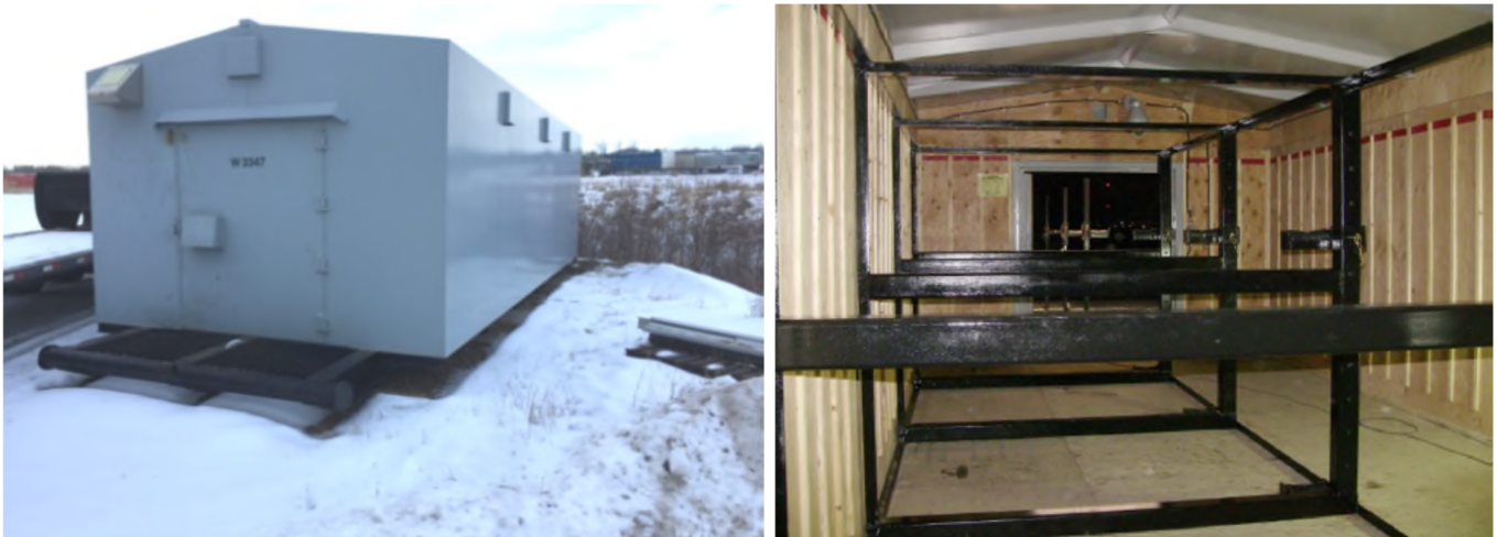
Figure 7. Additional Storage (Type 4 Magazine)
