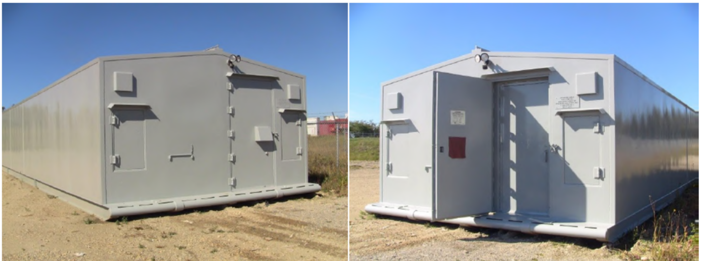
Figure 5. Standard Gun Loading Facility
