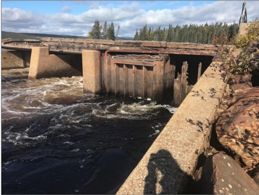
Figure B-1. Downstream end of fish ladder and spillway (10/09/2019)
