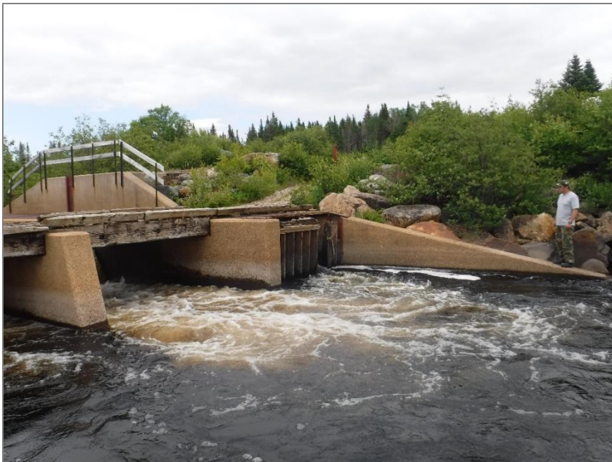
Figure B-2. Downstream end of spillway and fish ladder (07/14/2016)
