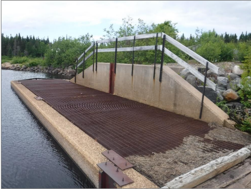
Figure B-5. Steel grating over fish ladder (07/14/2016)
