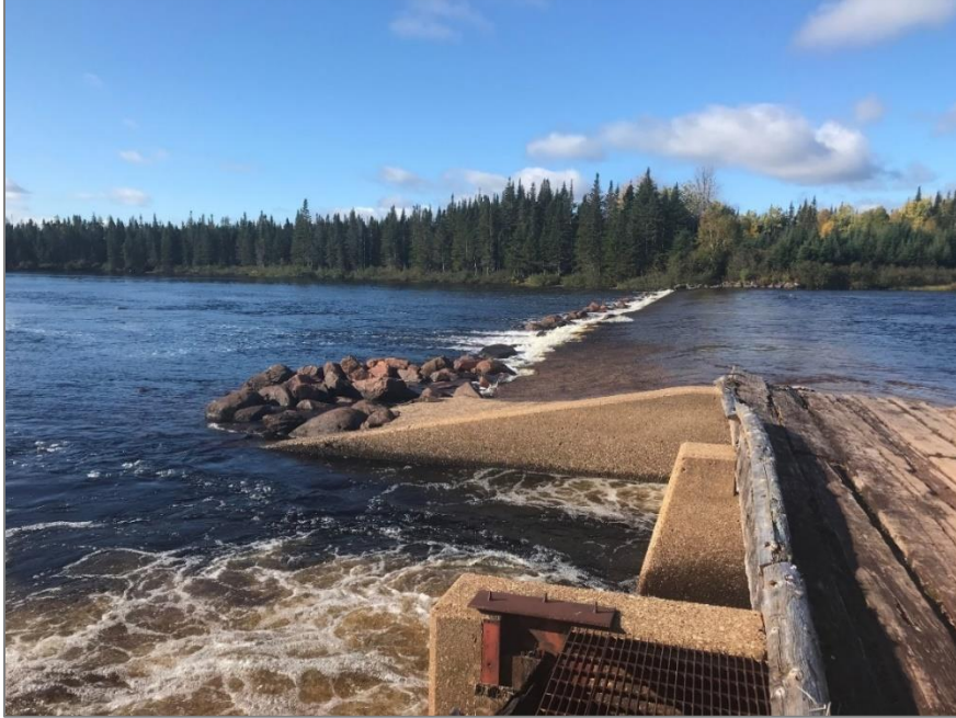
Figure B-7. Weir adjacent to project site (10/09/2019)
