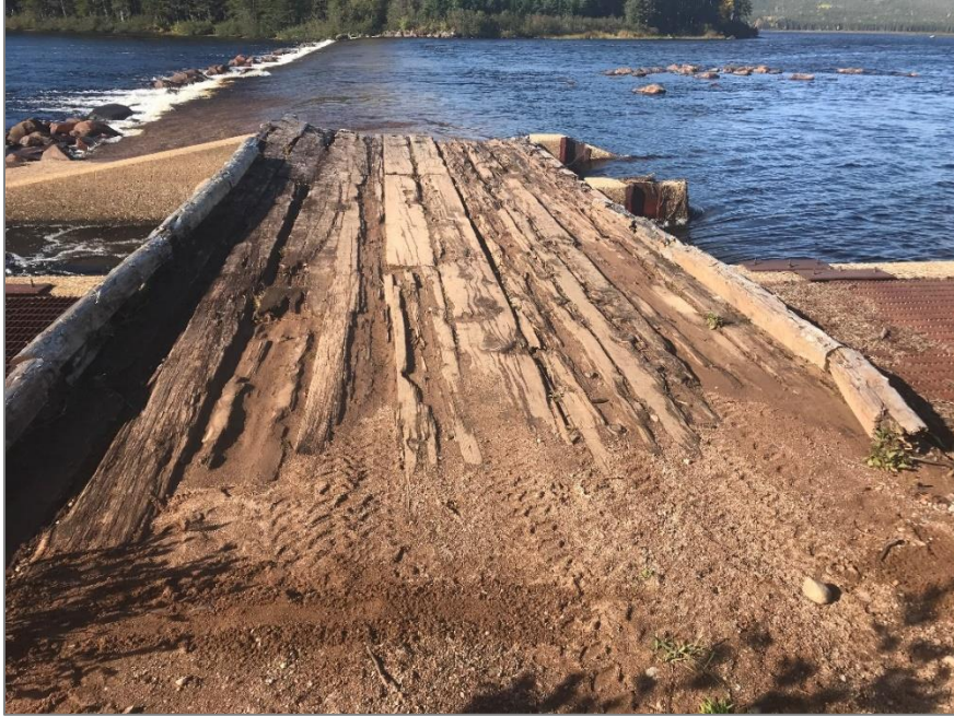
Figure B-3. Decking above fish ladder and spillway, adjacent to weir (10/09/2019)
