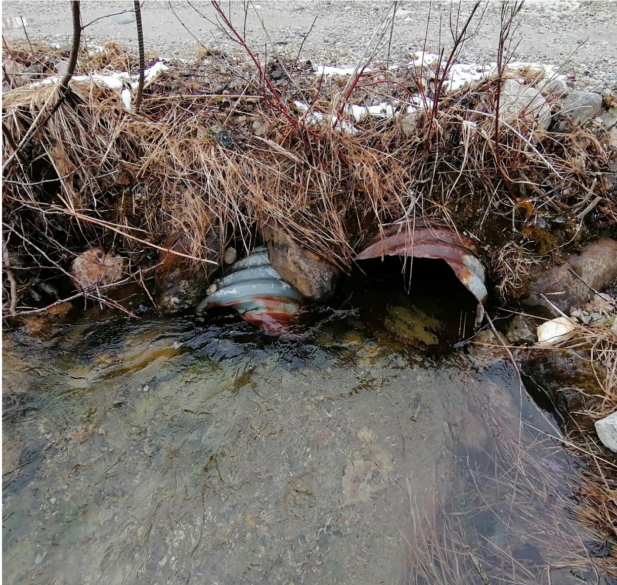
Figure 8: Existing 300mm and 450mm Culverts
