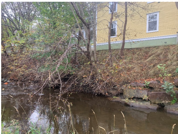
Photo 7: Armour stone wall erosion control improvements on south side of Rennies River across from tennis courts.
