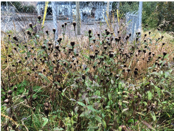
Photo 5: Berm 2 - Black knapweed ( Centaurea nigra ) and electrical substation.
