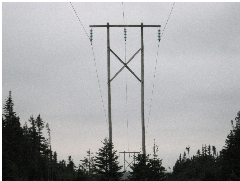
Figure 2-4 Photo of Typical H-Frame (Tangent) Structure
