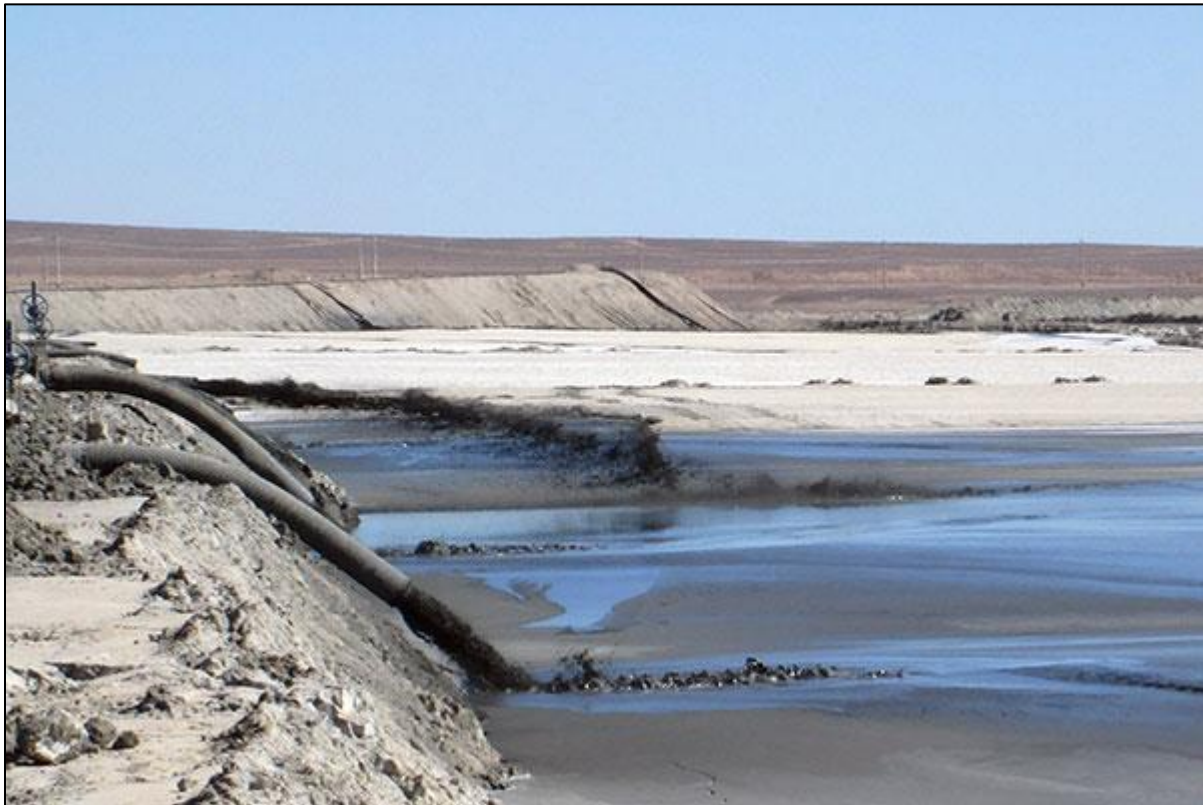
Figure 3.4 Photograph of Spigot Tailings Discharge.
