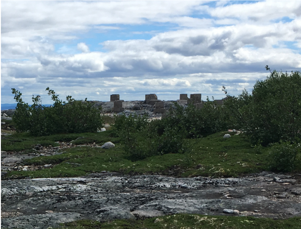
Photo 1 Upper Site: concrete foundation of former site structure. Looking south.
