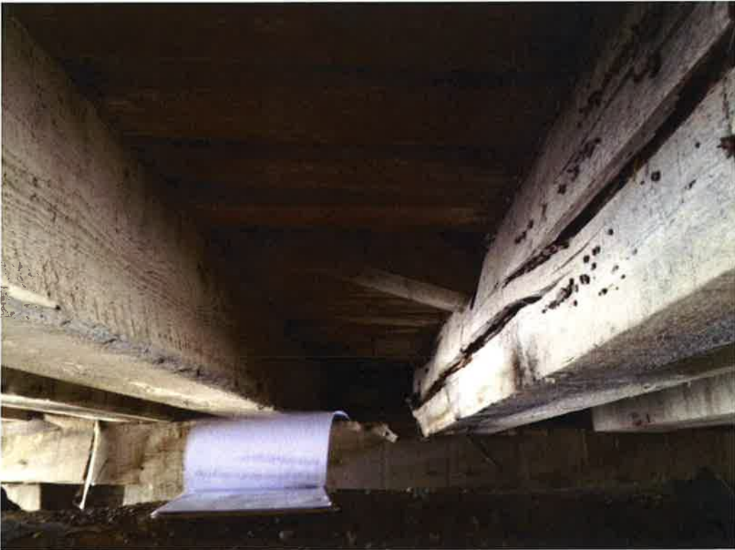
Gap between Beams 4 & 5 Looking South
