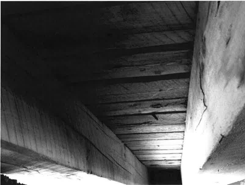
Gap between Beams 1 & 2 Looking North
