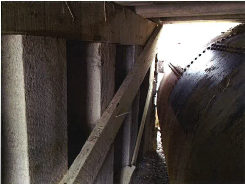
South Abutment Piles and Pile Cap
