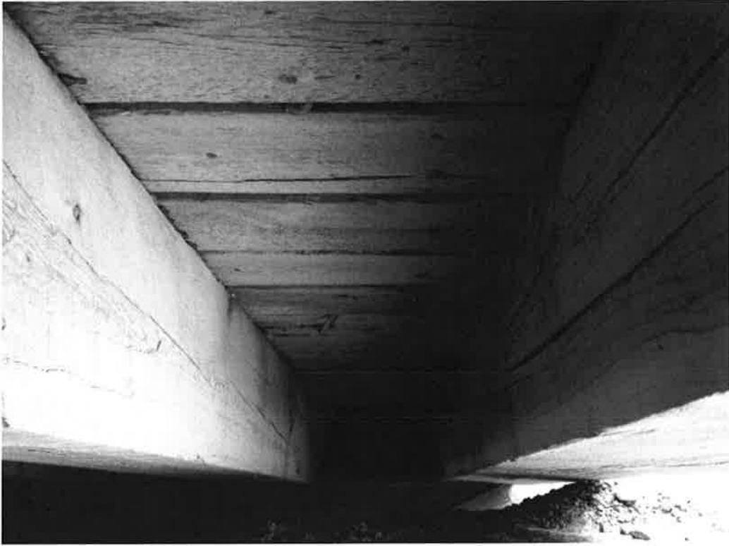
Gap between Beams 1 & 2 Looking South
