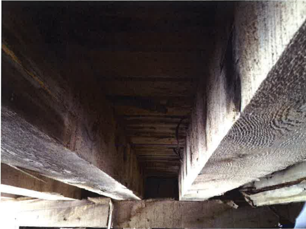
Gap between Beams 5 & 6 Looking South
