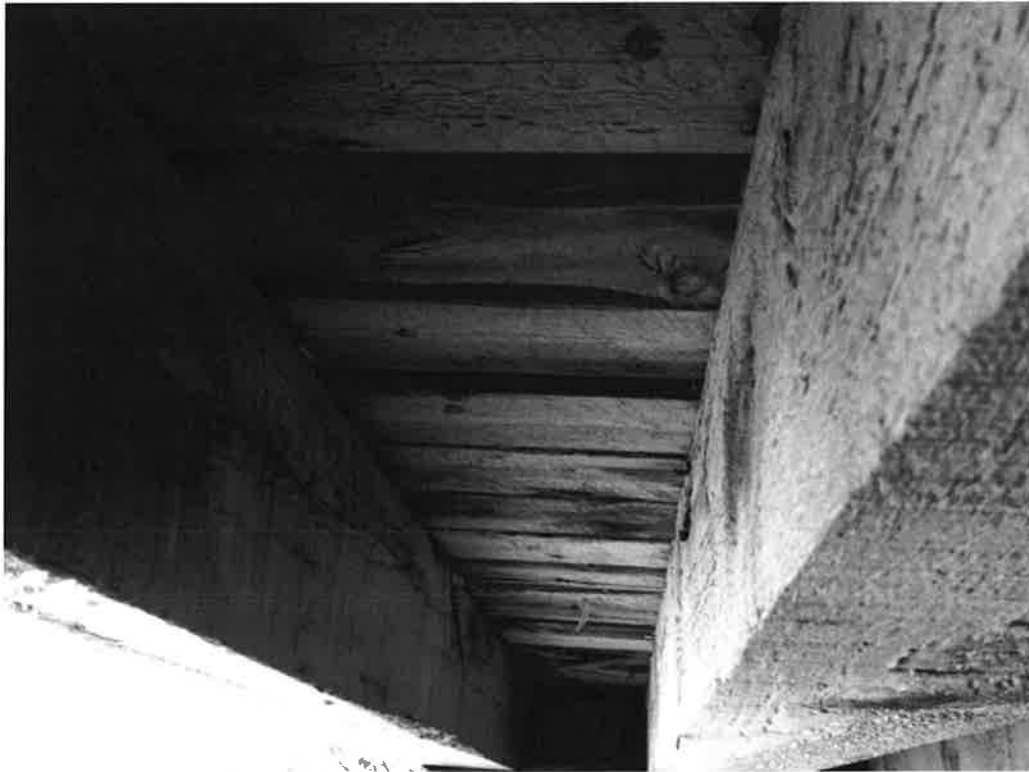
Gap between Beams 7 & 8 Looking South
