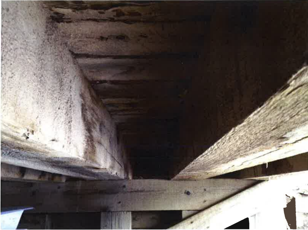
Gap between Beams 6 & 7 Looking North
