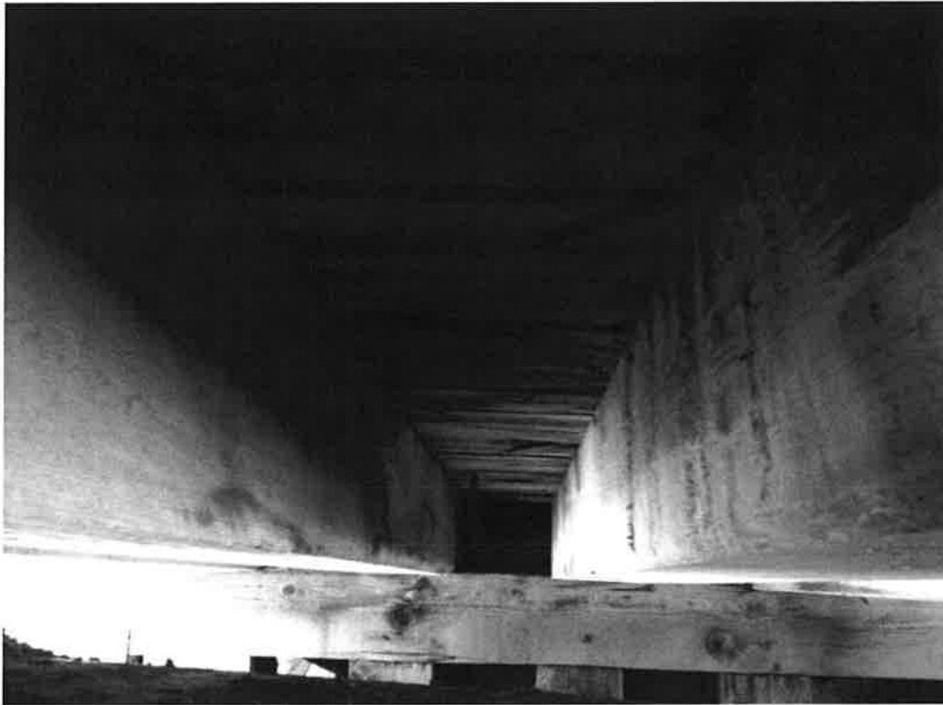
Gap between Beams 2 & 3 Looking North
