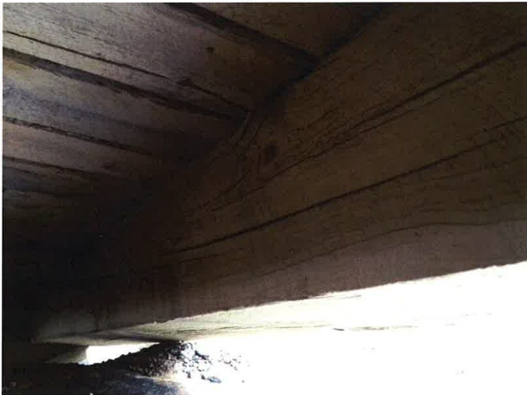
Longitudinal Splitting of End Beams
