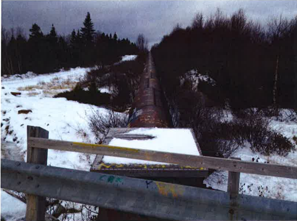
View from Bridge Looking West
