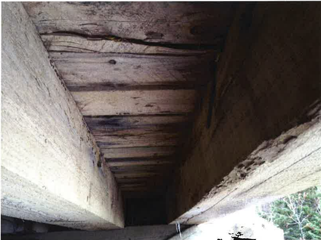
Gap between Beams 7 & 8 Looking North
