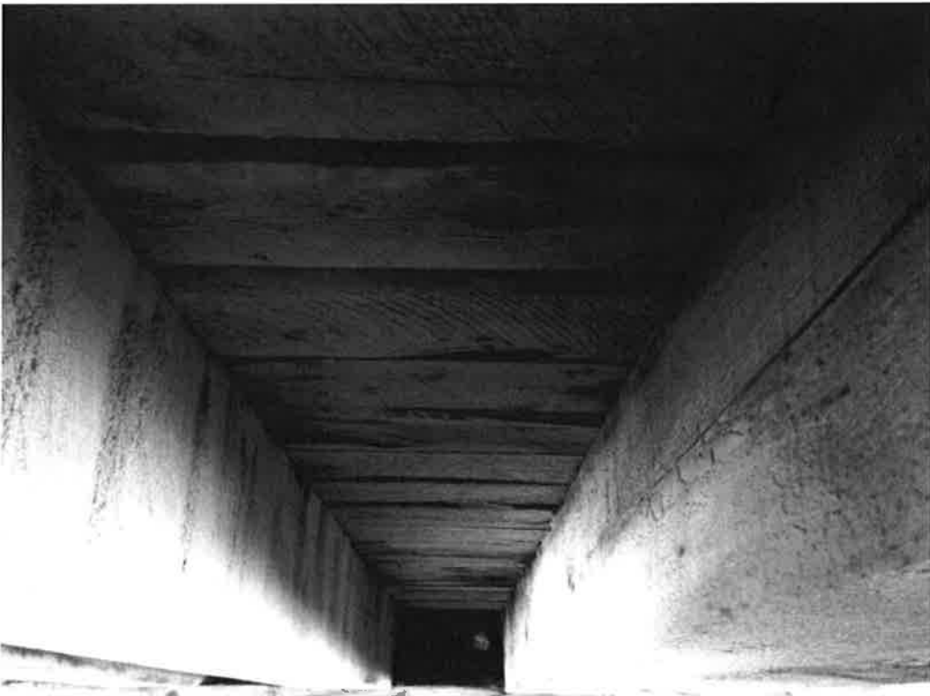
Gap between Beams 3 & 4 Looking North
