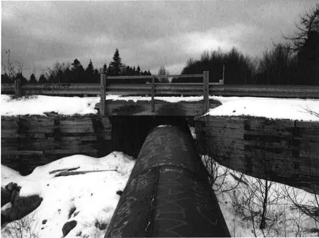
Bridge Looking West
