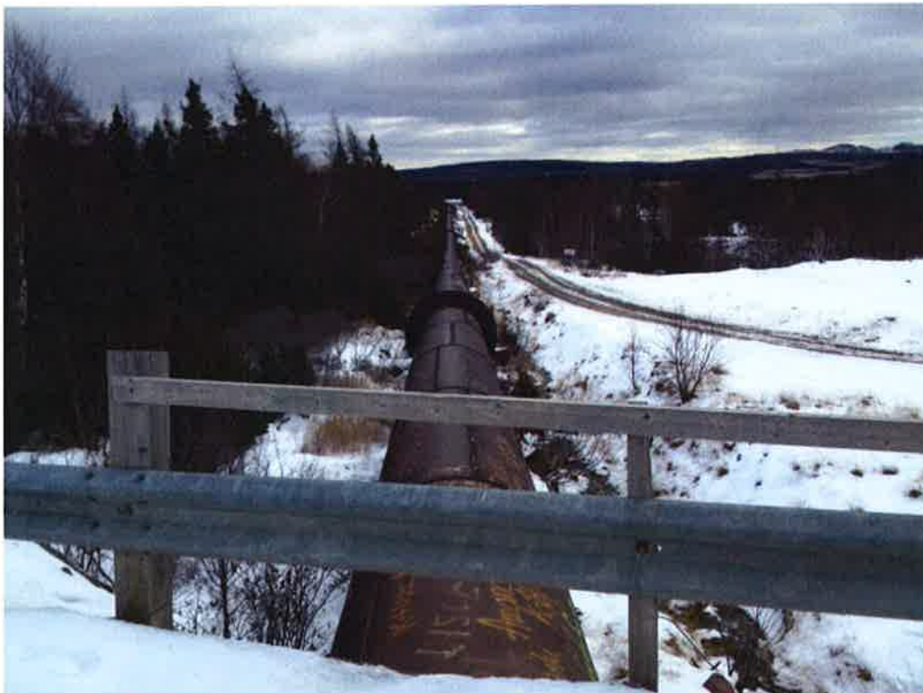
View from Bridge Looking East
