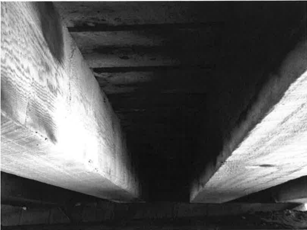
Gap between Beams 2 & 3 Looking South
