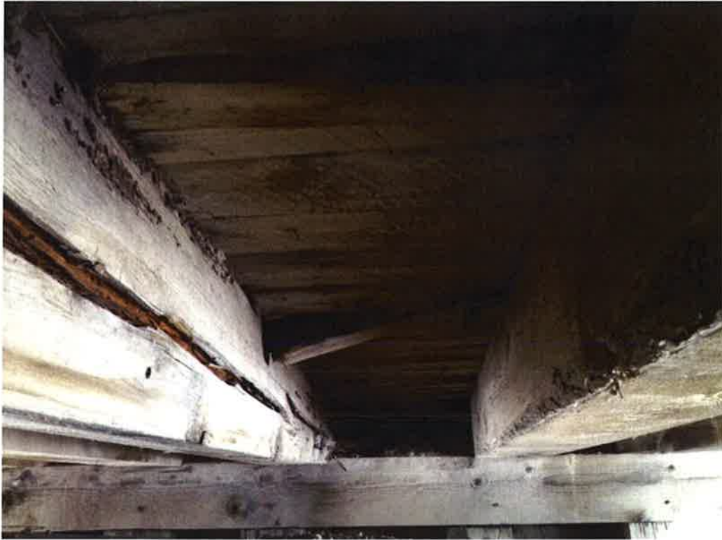
Gap between Beams 4 & 5 Looking North
