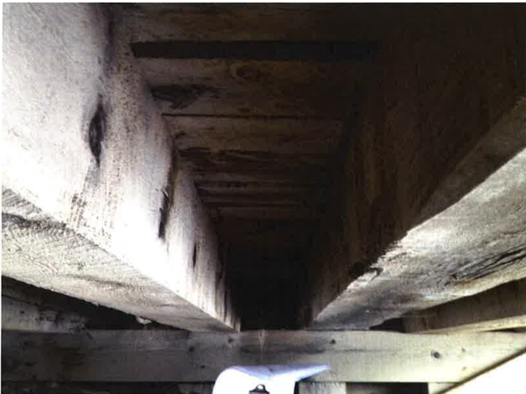
Gap between Beams 5 & 6 Looking North
