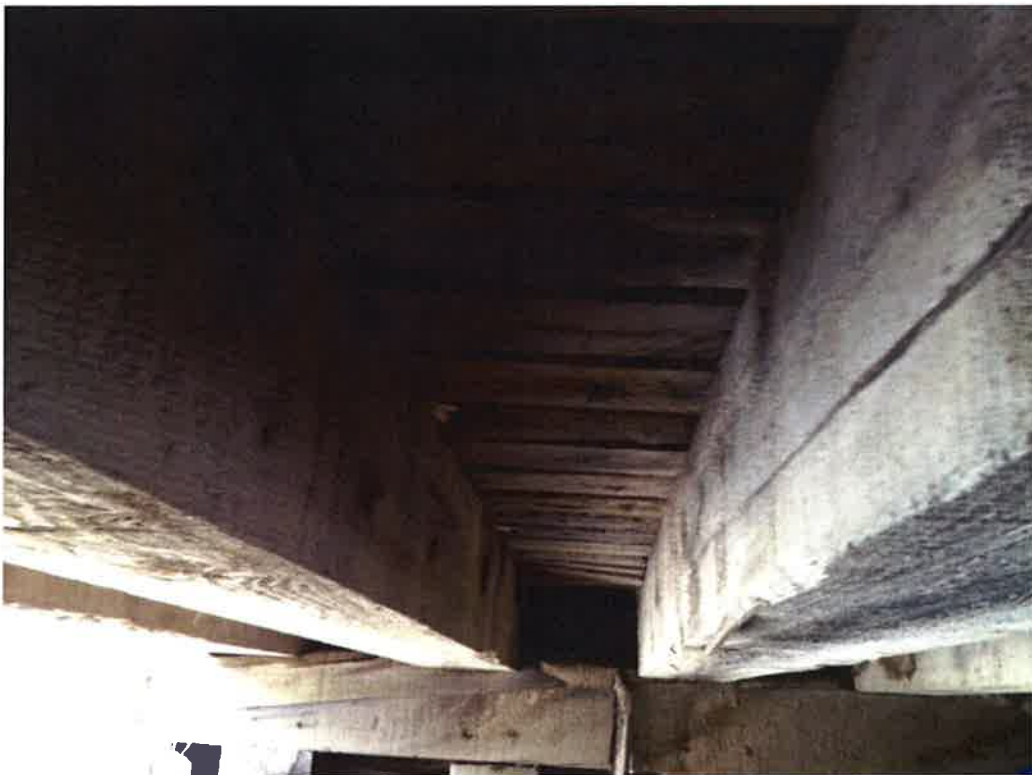
Gap between Beams 6 & 7 Looking South
