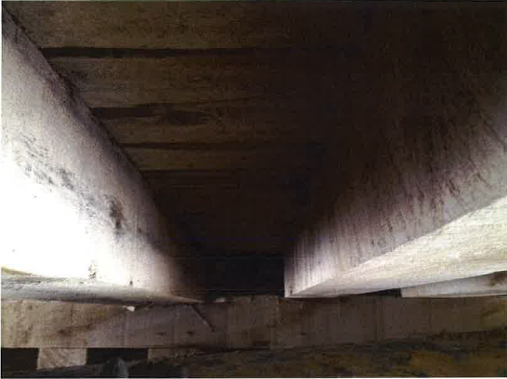
Gap between Beams 3 & 4 Looking South
