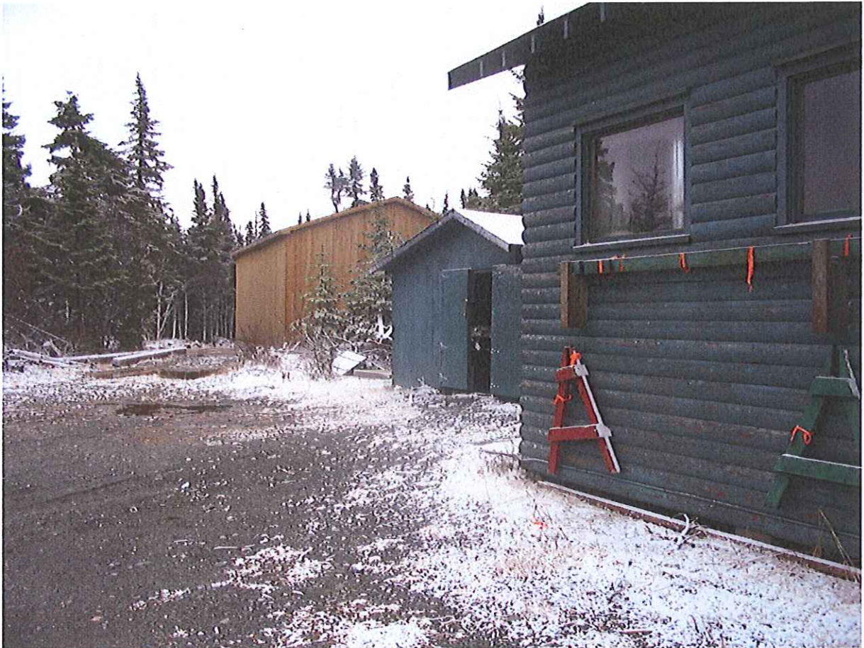
Photo#3: Looking southeast at shop, generator shed & garage from right to left.
