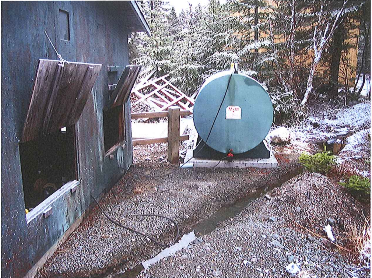
Photo#1: Looking southeast at back of generator shed. Note former AST & soil staining.
