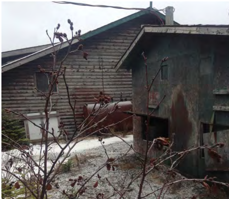
Photo 1 – View, looking northwest towards the generator shed and workshop during the December 2015 Site inspection.
