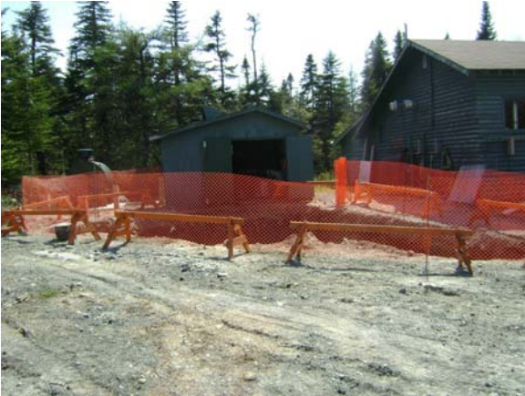
Photo 19: View of the barricades and snow fencing around the remedial excavation.
