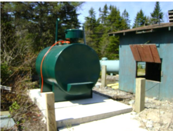
Photo 5: View of the 2,273 L diesel AST and the 2,000 lb (approx.) propane AST in background.
