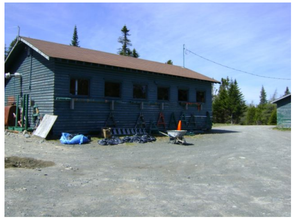
Photo 2: View of the north side of the workshop.
