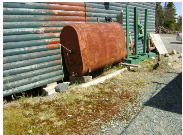
Photo 8: View of the 909 L heating oil AST.
