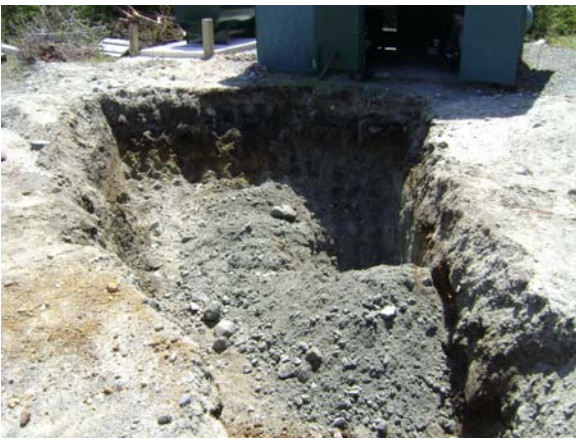
Photo 17: View of the soil conditions inside the remedial excavation.
