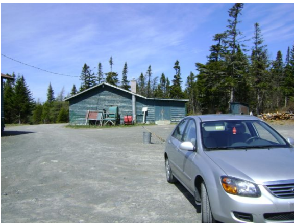
Photo 1: View of the east side of the water storage shed.
