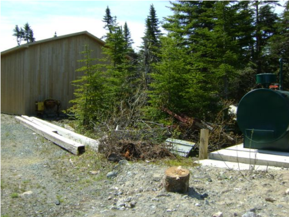
Photo 3: View of the west side of the groomer storage shed.
