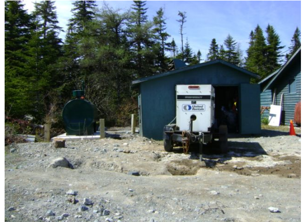
Photo 4: View of the north side of the generator shed.
