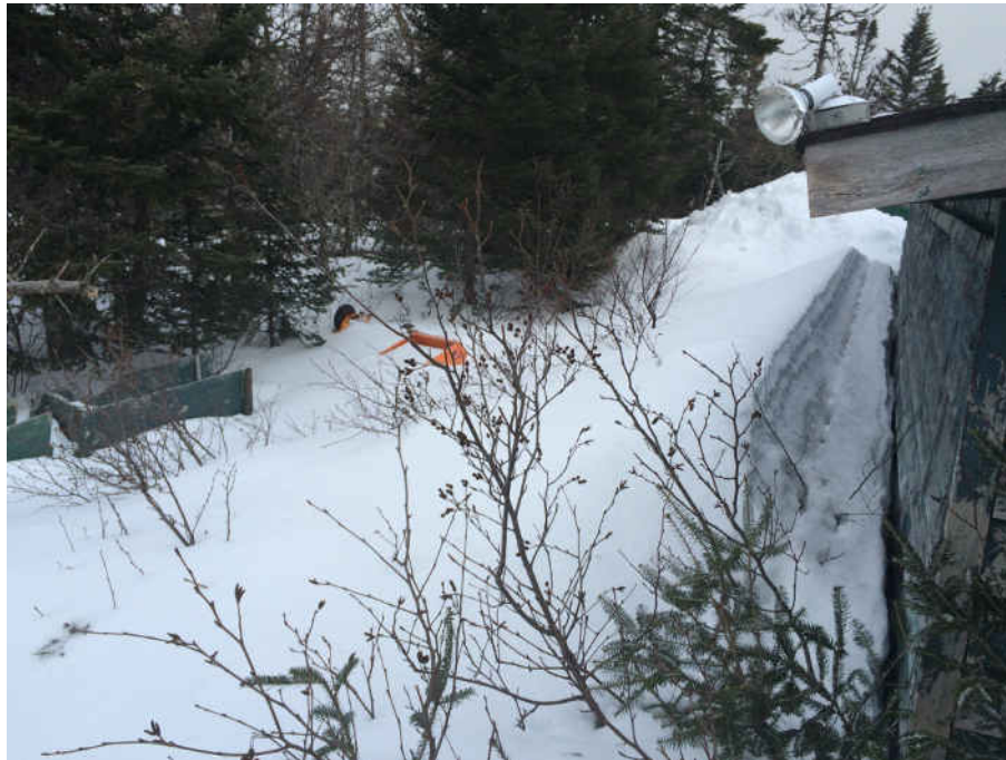
Photo 7: Trailers and building materials buried in the snow at proposed sampling area.
