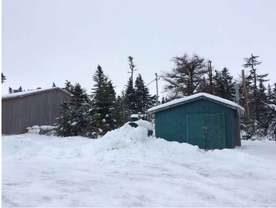
Photo 1: View of the storage shed (Left), diesel fuel tank and generator shed.
