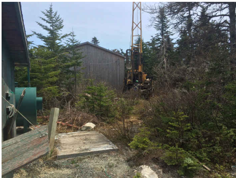
Photo 10: Monitoring Well MW-3 Installation.
