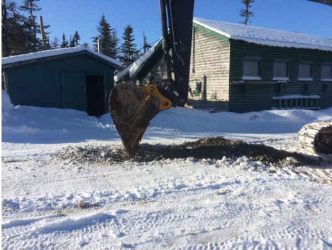
Location of Test Pit 1.
