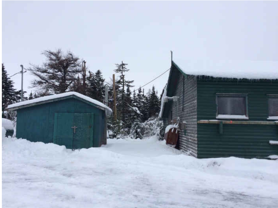
Photo 2: View of generator shed (Left) and workshop (Right).
