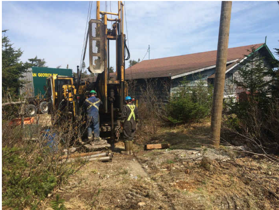
Photo 11: Monitoring Well MW-4 Installation.
