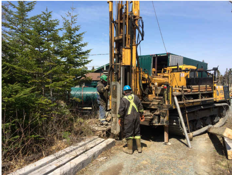
Photo 9: Monitoring Well MW-2 Installation.
