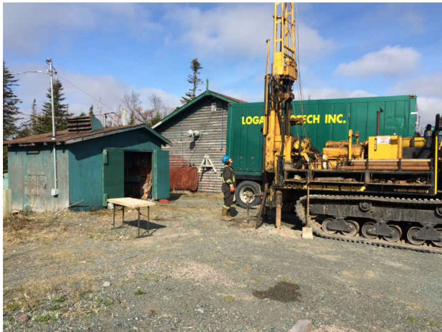
Photo 8: Monitoring Well MW-1 Installation.
