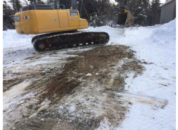
Test Pit 1 after being backfilled.
